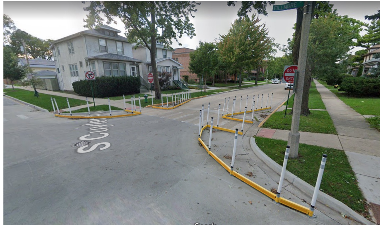
Bump-Out @ Irving Elementary Cuyler Ave. and Fillmore St.
