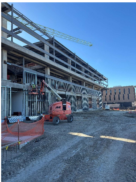
North Elevation – Exterior Stud Framing
