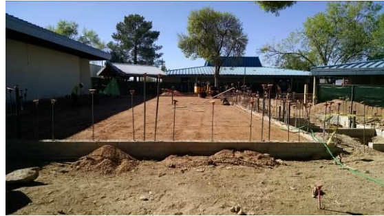
Preparing for Concrete Pad at New Building
