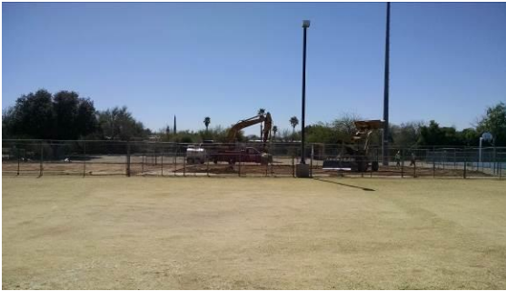
Grading old portable area
