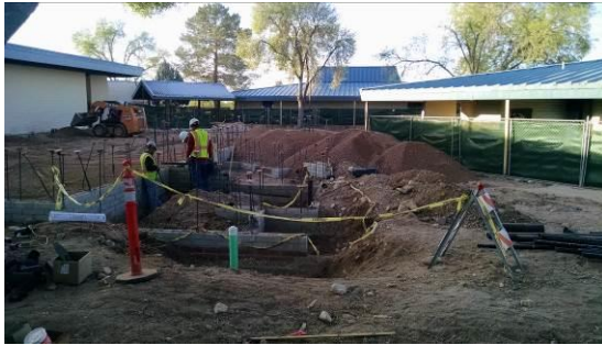
Preparing for Concrete Pad at New Building
