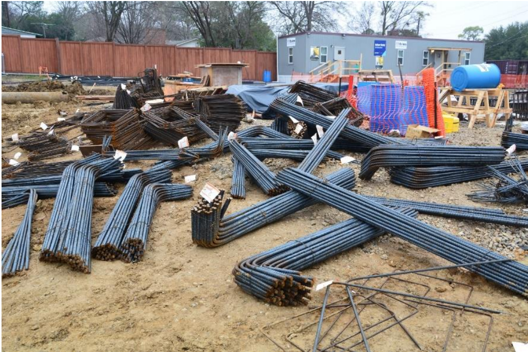
Grade beam reinforcement material is on site.
