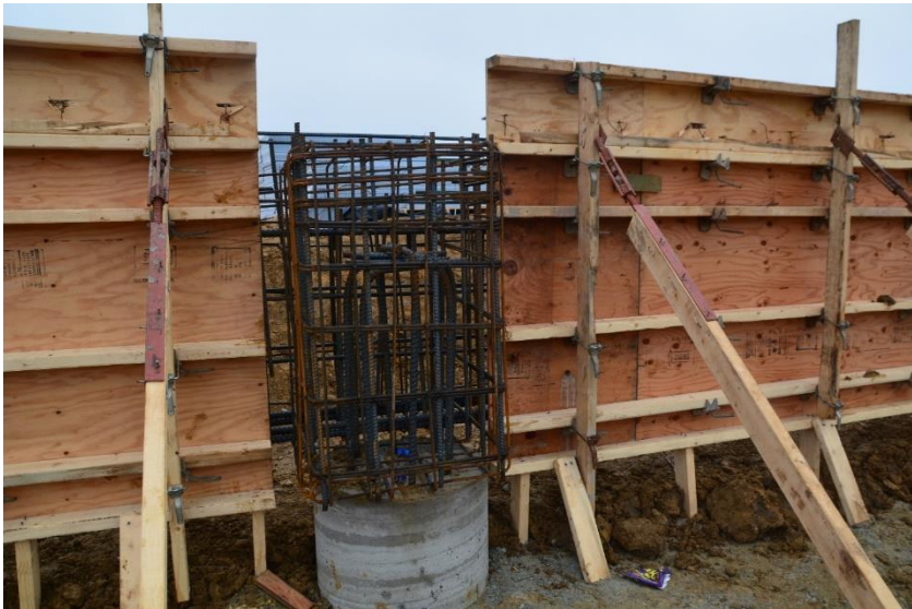
Reinforcement steel above pier in grade beam
