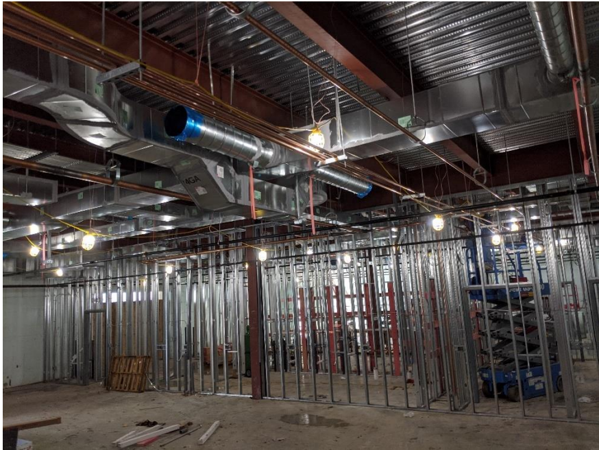
Interior Framing for Storm Shelter
