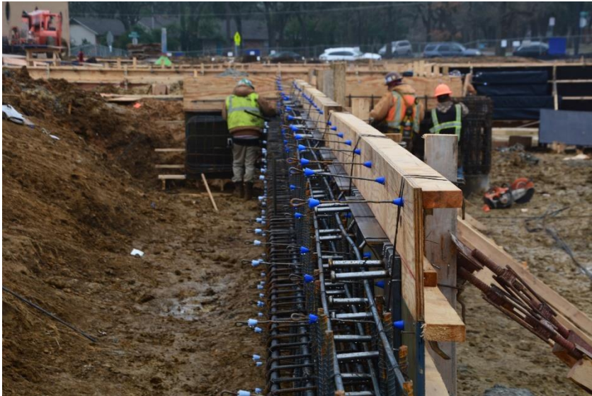
Reinforcement steel is being placed in the grade beams.
