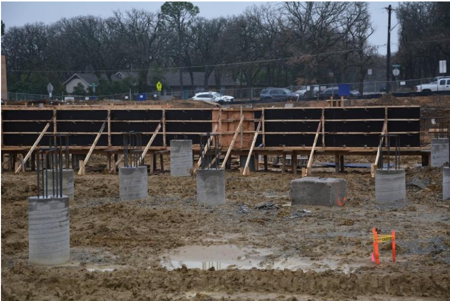
Formwork for grade beams has begun.
