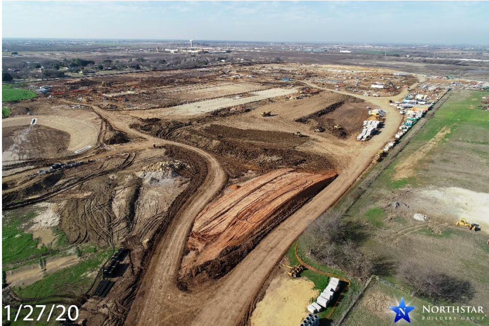
Looking Southeast to Northwest.
