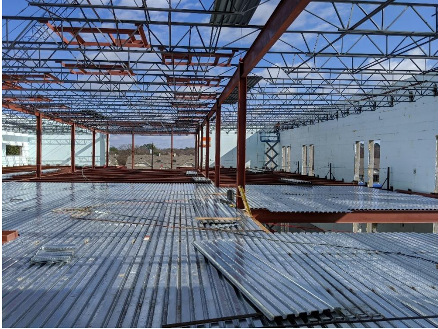
Area A Steel, Joist, and Decking
