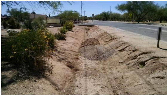
Ditches and pipes
