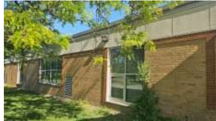
Exterior – New Windows & Louvers
