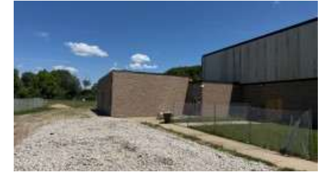
Exterior – Classroom Addition
