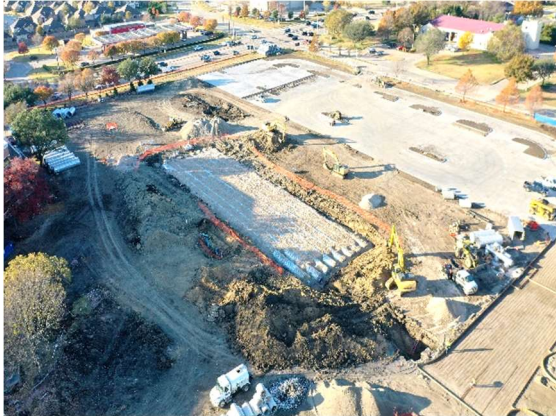
Aerial of Site - Phase 2 Work
