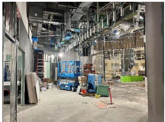
Serving and Seating Area at Kitchen Renovations
