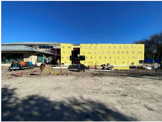
Sheathing Installed at Dining Hall Addition
