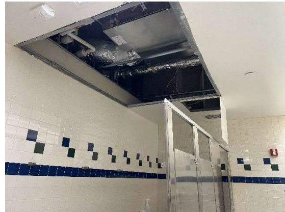
Fan Powered Box Install at Heritage Hall
