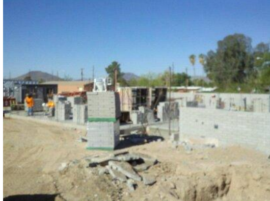
exterior block walls
