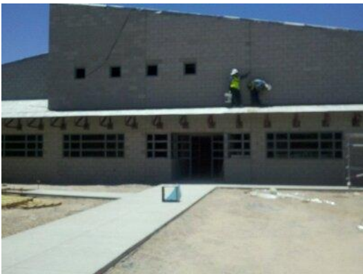
front entrance to Rillito Center
