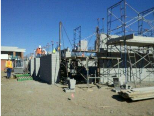
Exterior CMU wall installation MRR demo and new kitchen / serving line work
