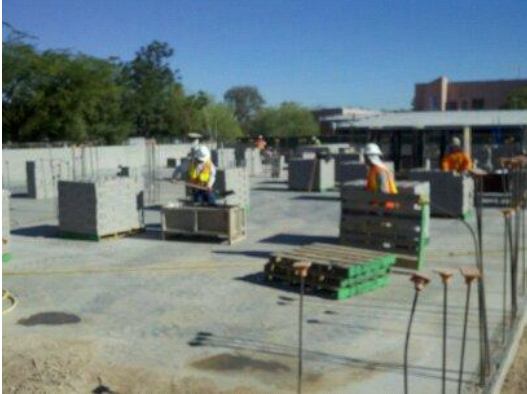
new building S.O.G.
