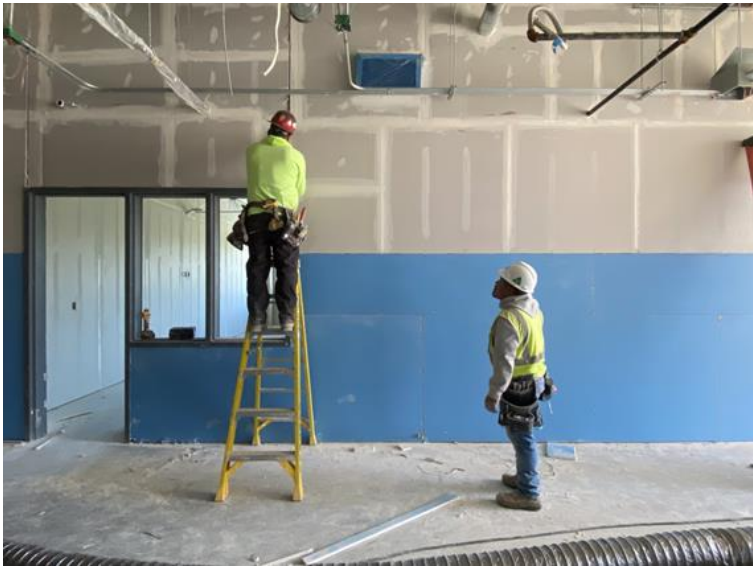
Installing Drywall Joints on 1 st Level
