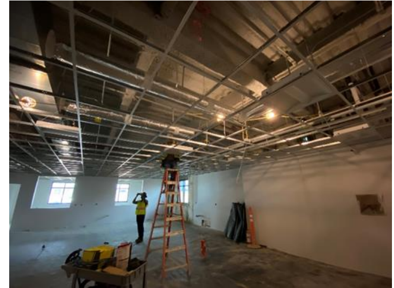
Installing Light Fixtures in Area 1
