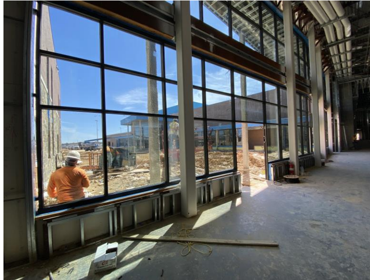
Installing Storefront in Area 3
