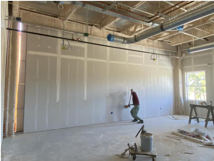
Finishing Drywall on 2 nd Level
