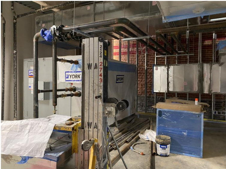
Air Handling Unit on 1 st Level
