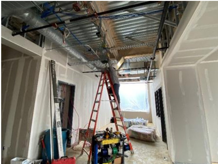
Installing Overhead MEP on 1 st Level
