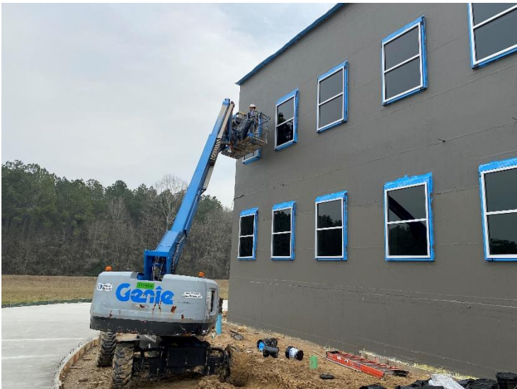
Installing Exterior Windows
