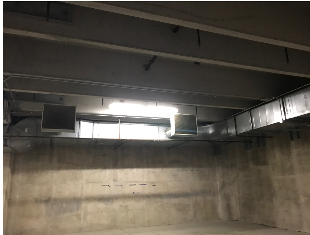
EAST WALL PHOTO 2
