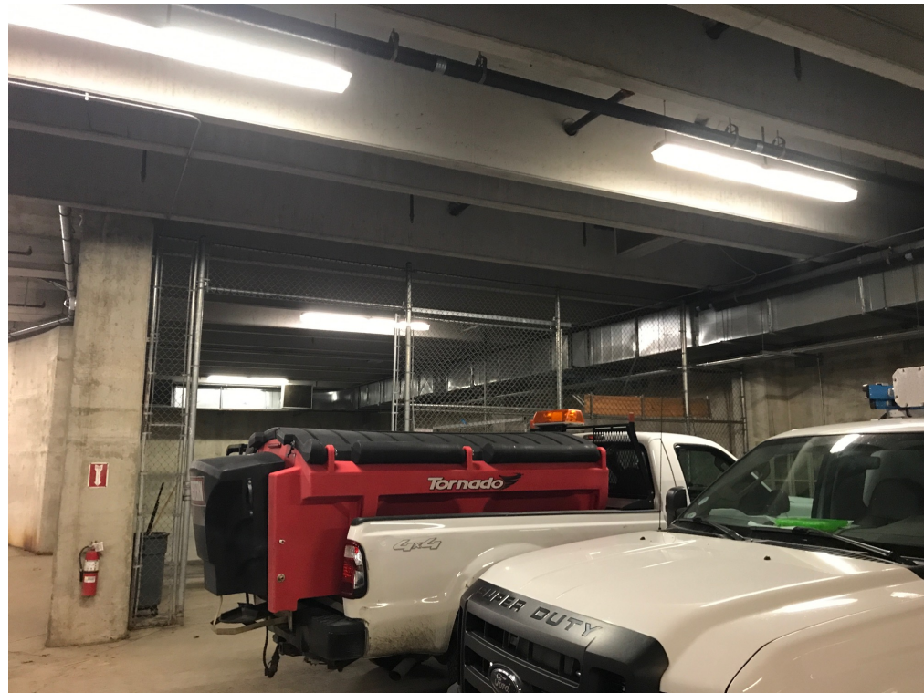
PHOTO AT SOUTH WALL AT EAST END OF D97 AREA
