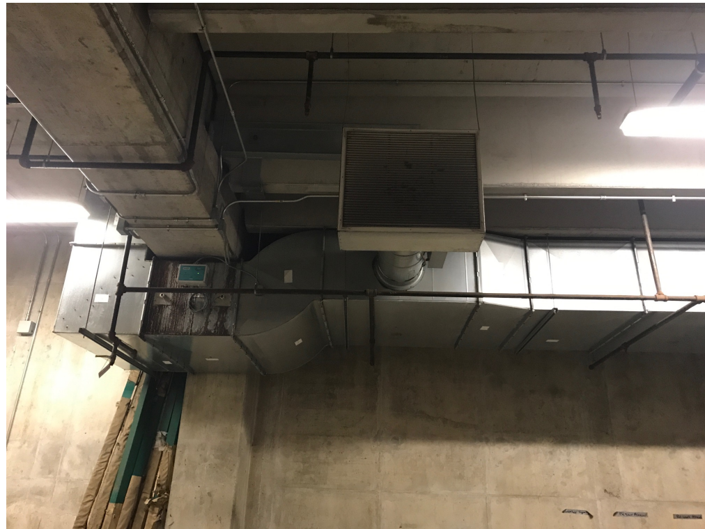
EAST WALL PHOTO 1
