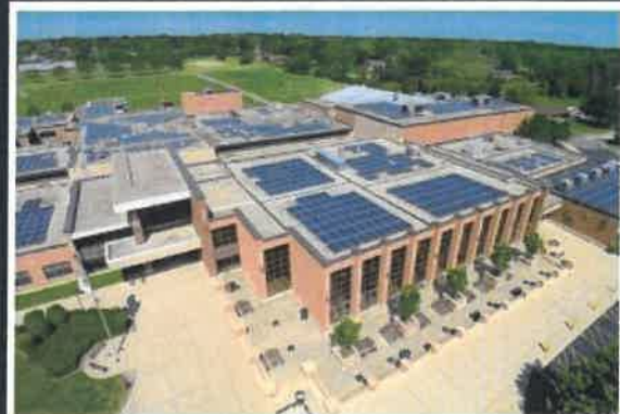
Lake Park HS Solar Installation Example
