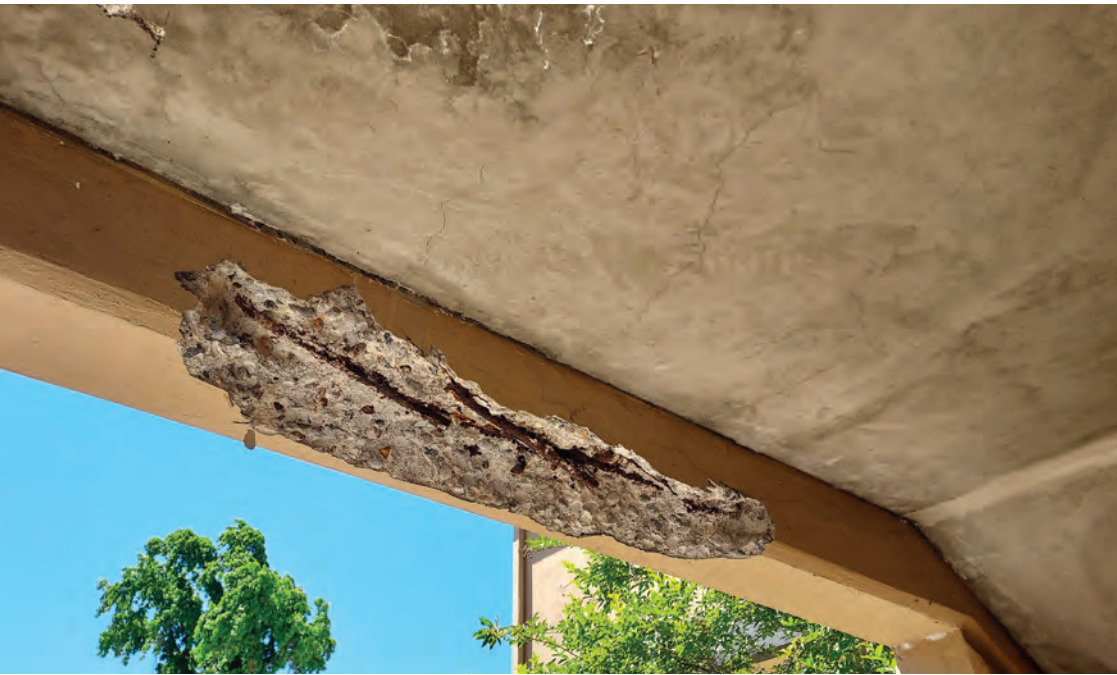
1 (STL) CORROSION OF (E) STEEL STRUCTURE
