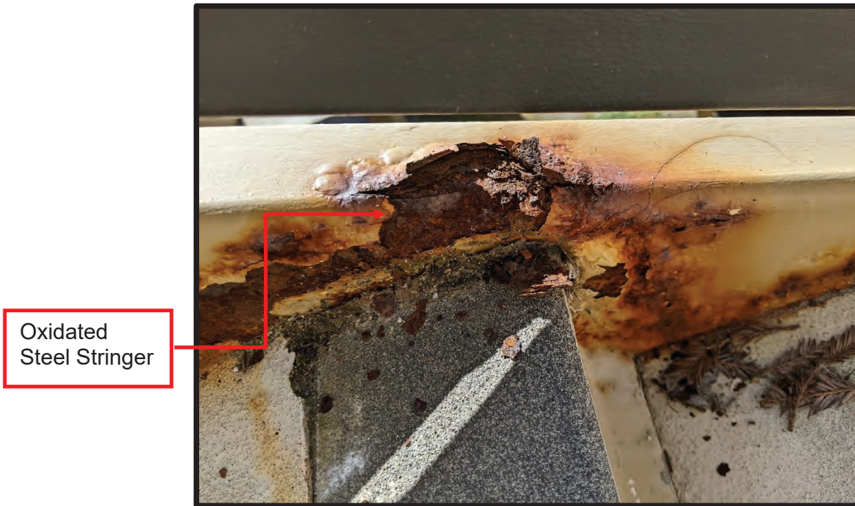
Photo 9: North-West Tube Steel Stringer
