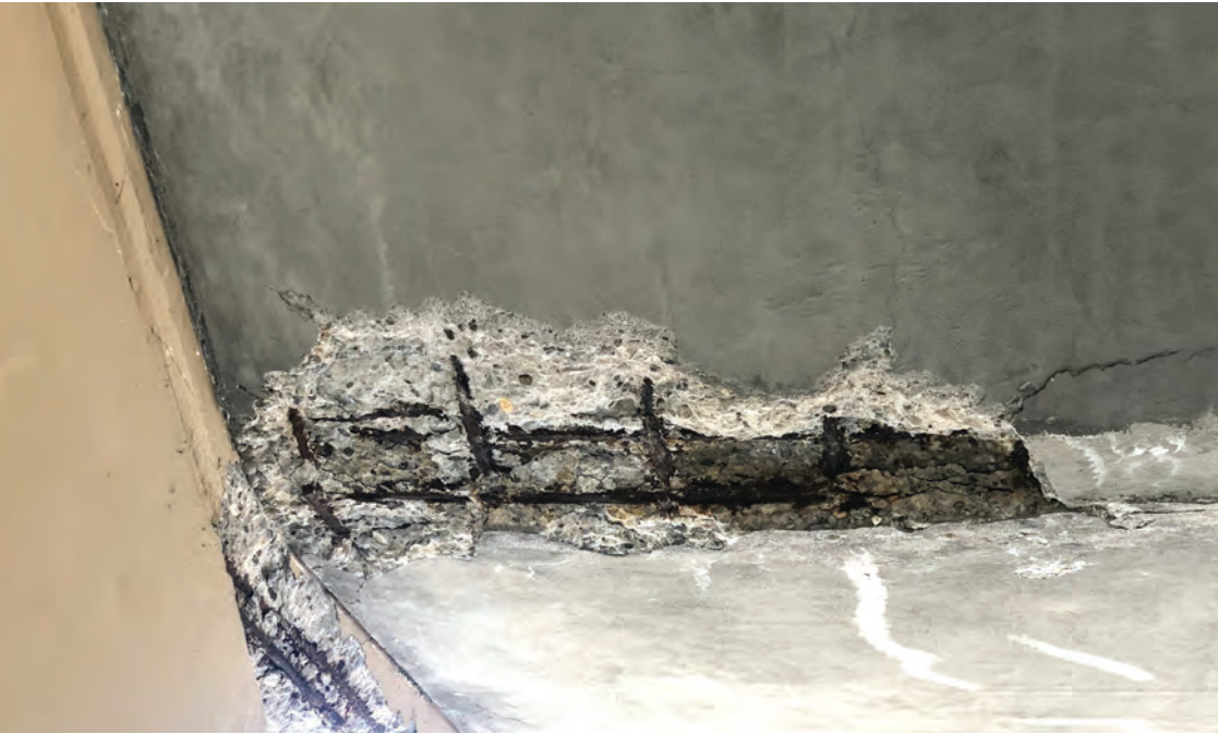
4 STL CORROSION OF (E) STEEL STRUCTURE
