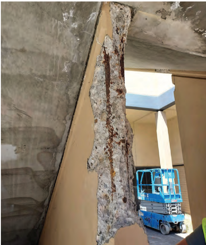
2 (STL) CORROSION OF (E) STEEL STRUCTURE
