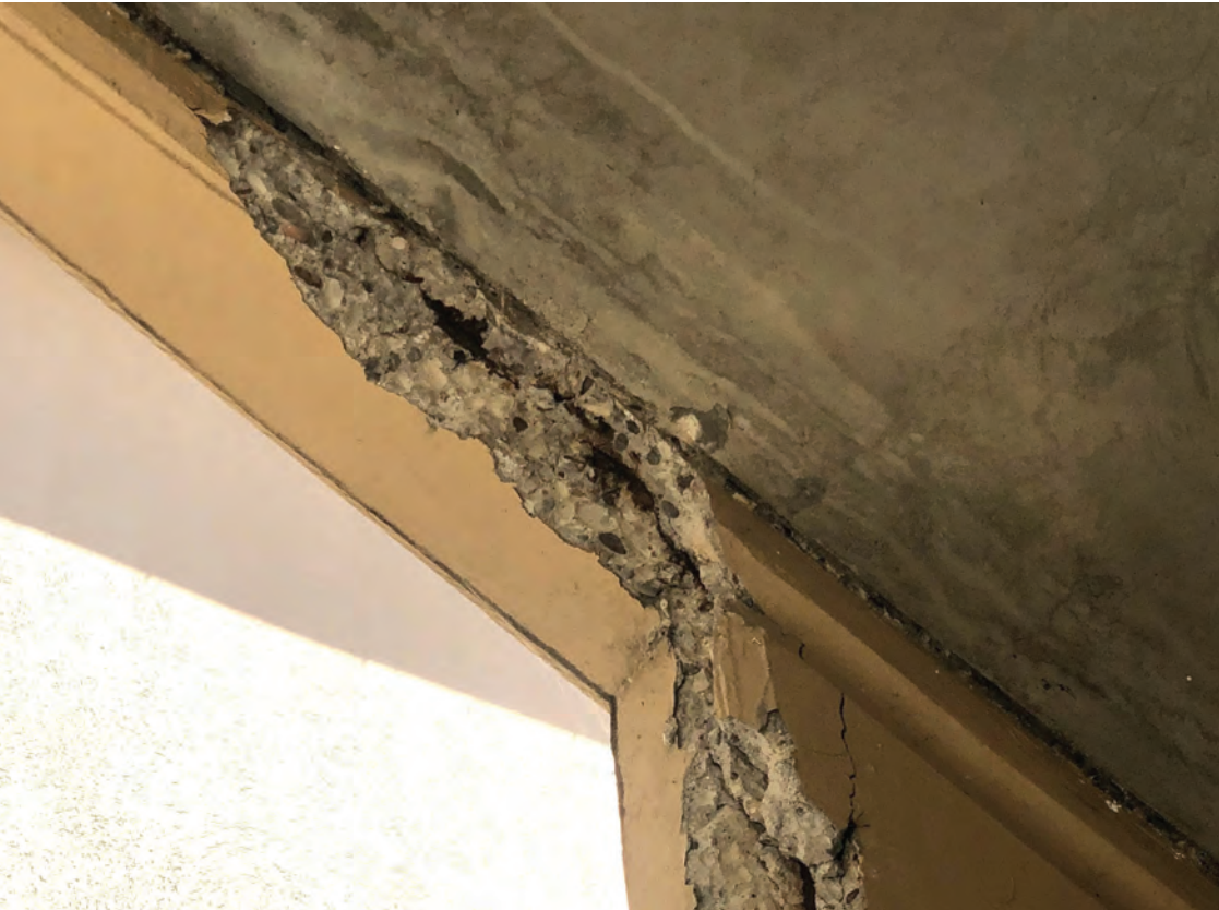
6 STL CORROSION OF (E) STEEL STRUCTURE
