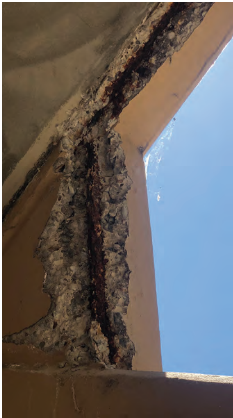
5 STL CORROSION OF (E) STEEL STRUCTURE
