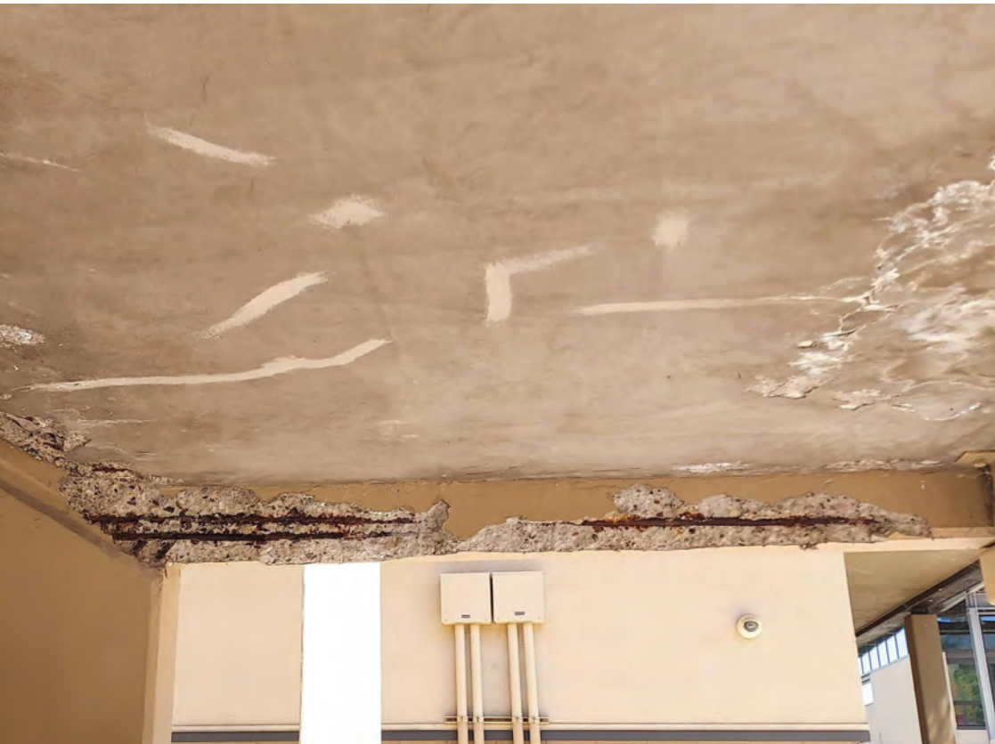
3 (STL) CORROSION OF (E) STEEL STRUCTURE
