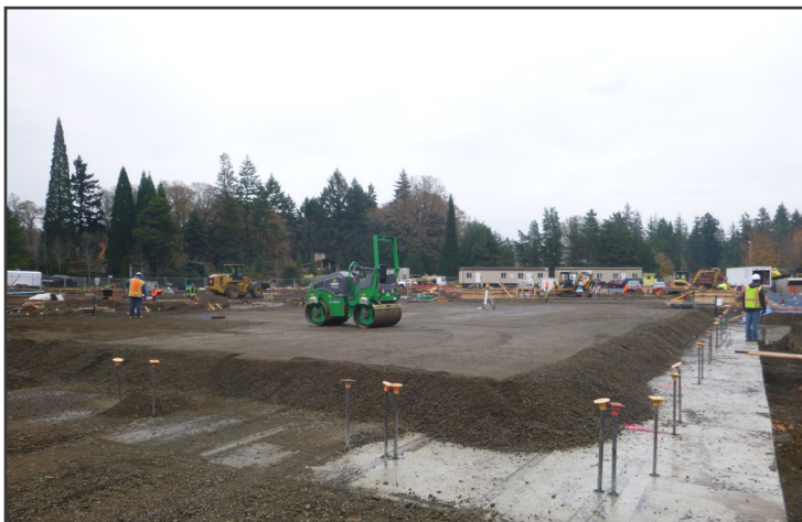
Concrete slab preparation for gym
