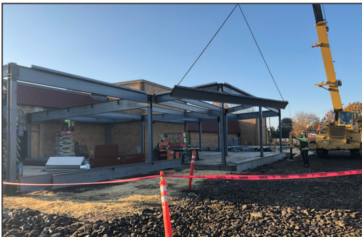
Structural steel installation
