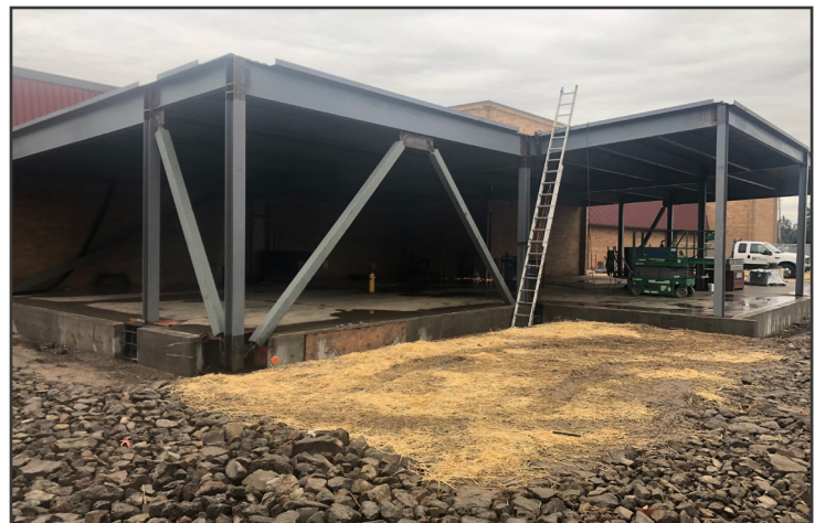
Roof decking on new addition
