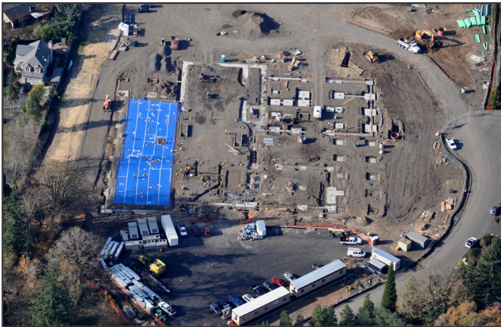
Aerial looking west
