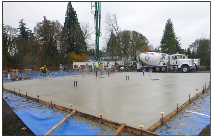
Concrete slab in Admin. Office and SPED area
