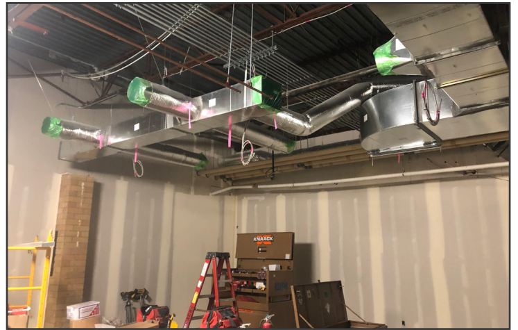
Classroom HVAC rough-in
