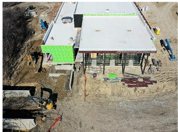
South View of Conference Center
