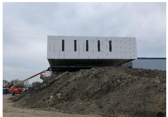
Swiss Pearl Installed on South Truss at Academic Building
