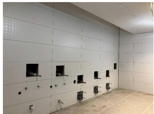
Restroom Tile Installed at Campus Commons
