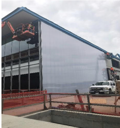
Polycarbonate Install on South Side of Trade Bar B
