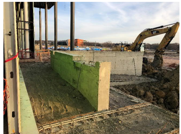
Retaining Wall Outside of Conference Center
