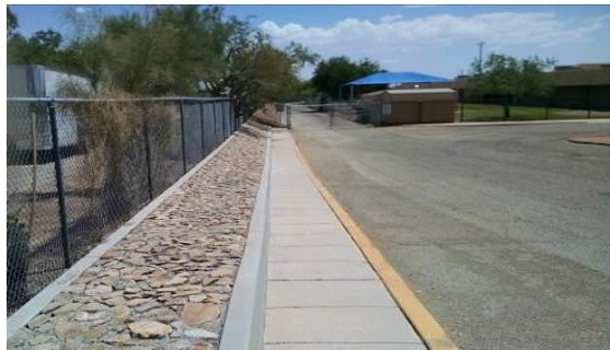
New rip-rap along east property line
