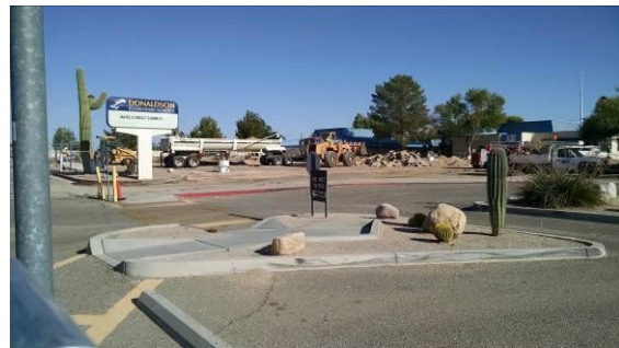
Bus Loop Demolition
