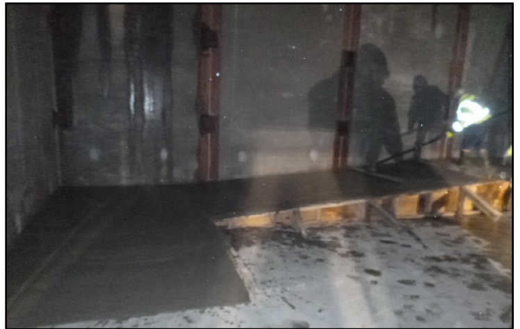
Freshly placed concrete
