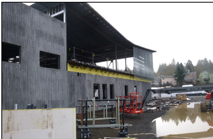
West facade of building
