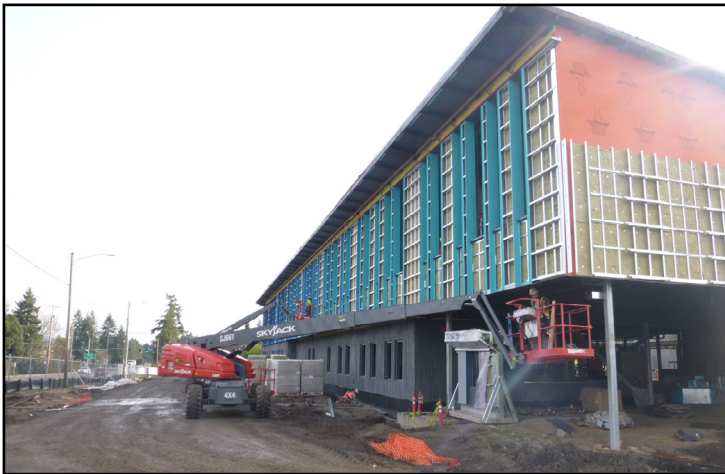
North facade of building
