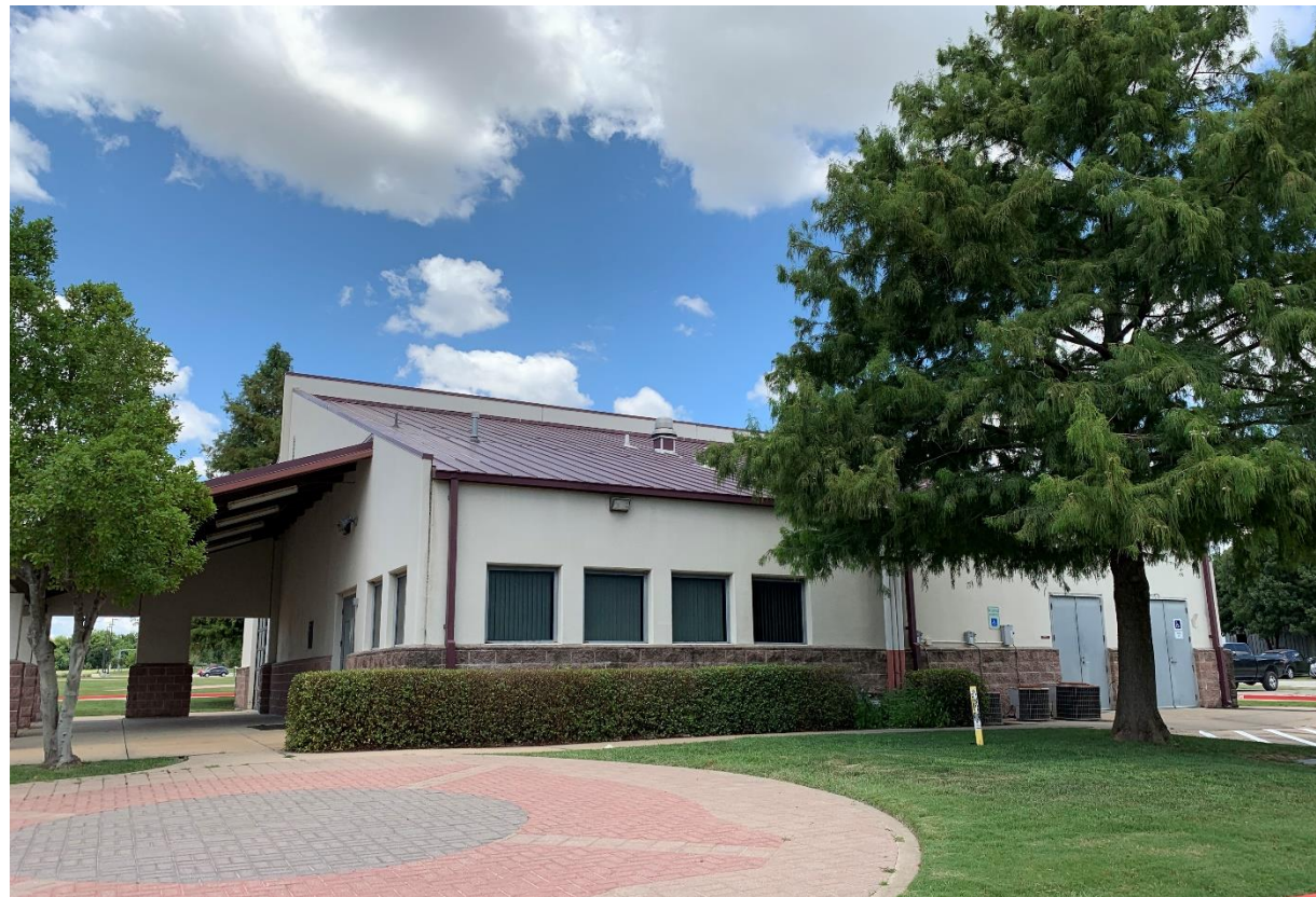
FIELD TRAINING BUILDING
