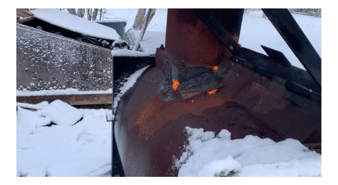
Rotted pipe nipple in heating system:
