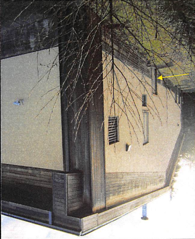
HCSHMG Rear view. Portion of horizontal wooden base is buckling. Investigating reason(s) why. Recommend
