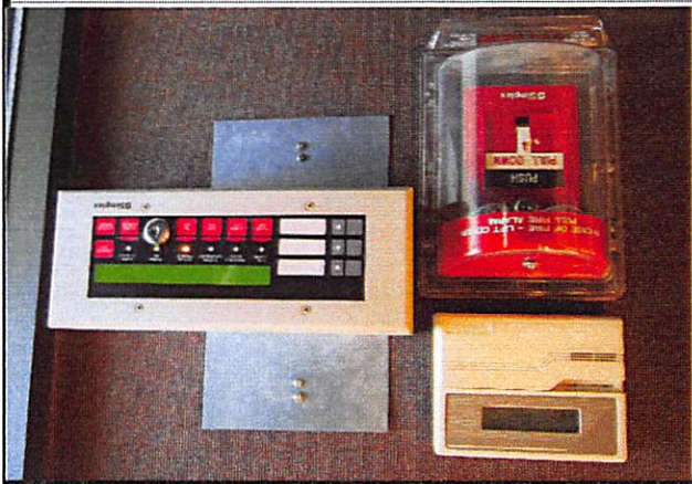
HCSJSHS Simplex Fire Alarm panel reported a "trouble" condition at the time of the site visit.
