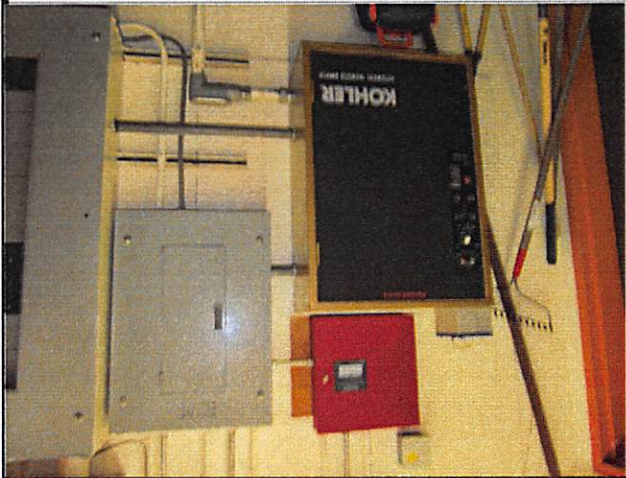
HCSJSHS Simplex Fire Alarm panel reported a "trouble" condition at the time of the site visit.
