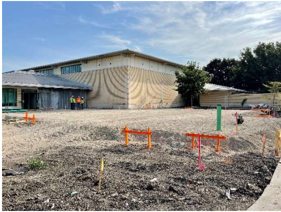
Building Pad for Kitchen Additions
