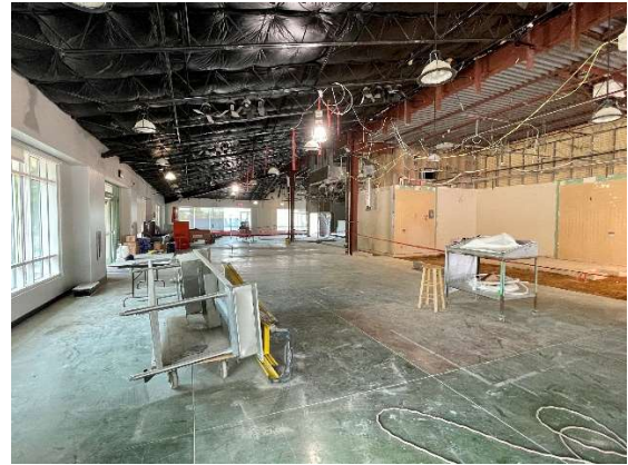
Interior Renovation in Dining Hall
