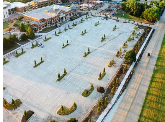
North Parking Lot Complete
