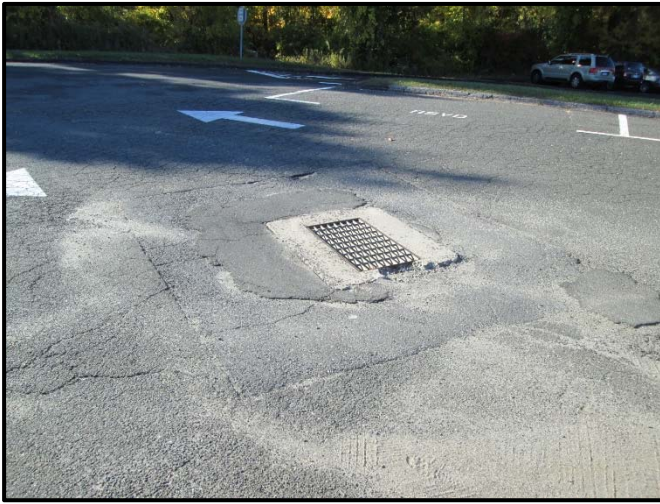
Catch basin beginning to deteriorate.
