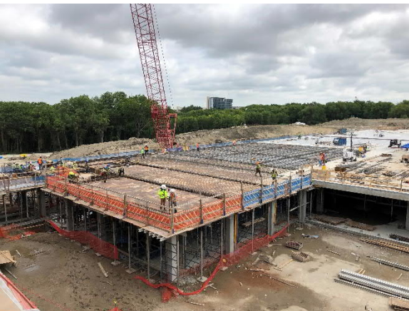
Garage – Elevated Deck Pour at Building D
