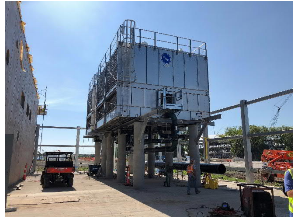
Central Utility Plant – Cooling Towers
