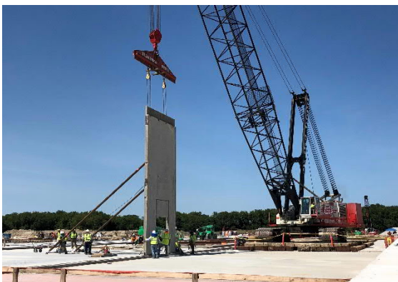
Building B – 1 st Panel Erection
