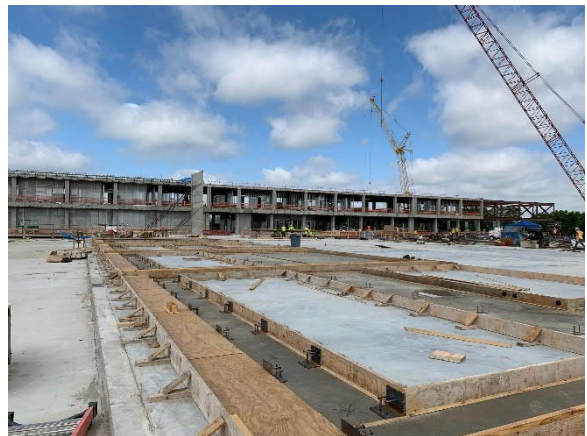
Building C – Tilt Wall Panel Forms
