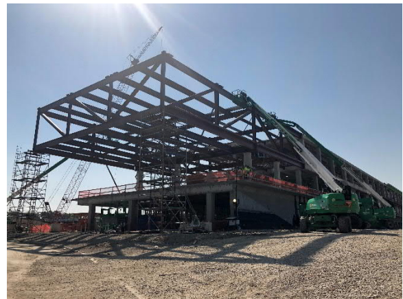
Building A – North Truss
