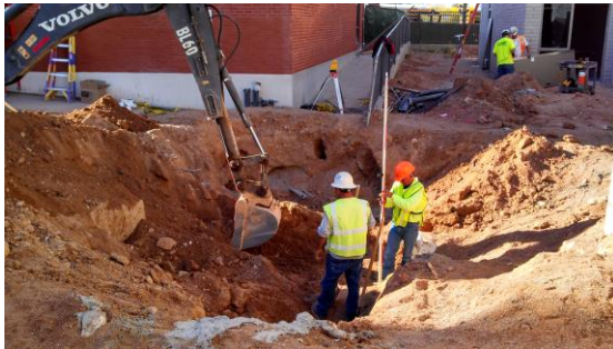
Storm Water Evacuation Improvements
