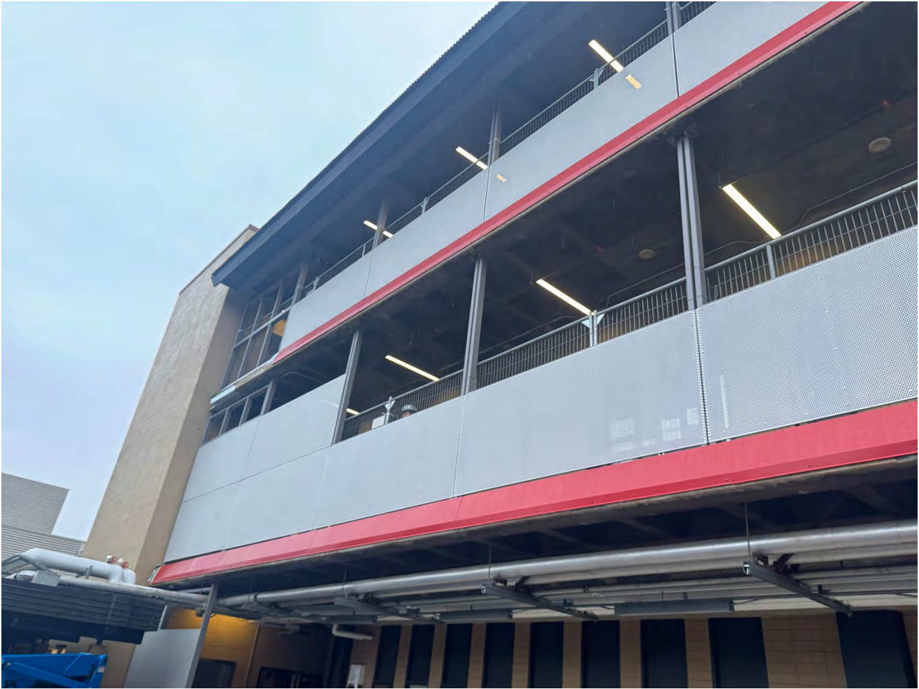
New Humanities Building Safety Railing
