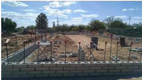
Walls being constructed for new classrooms
