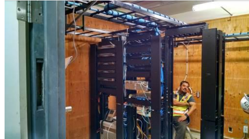
New IDF room addition
