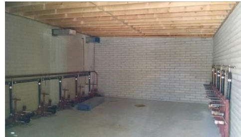
Library restroom renovation
