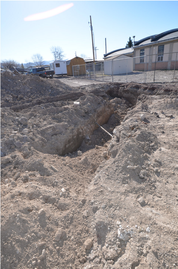
01 - Sewer Line Excavation.JPG
