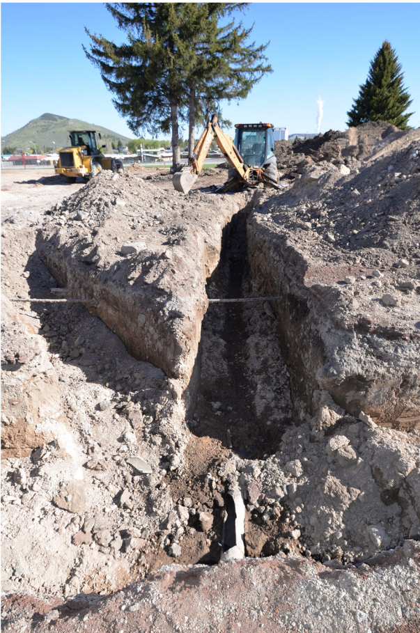
03 - Sewer Line Excavation.JPG
