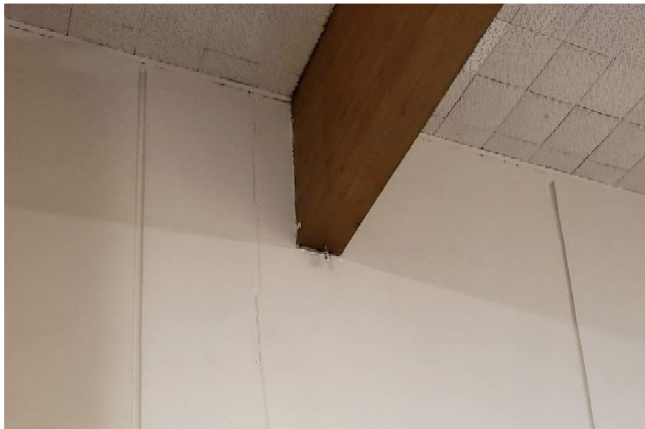
Figure 4: Crack in exterior concrete wall
