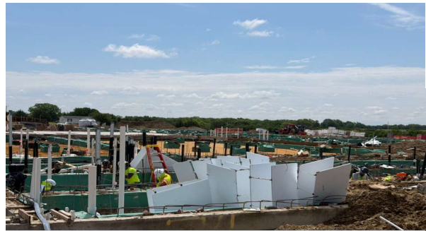
FOUNDATION & UNDERGROUND UTILITIES
