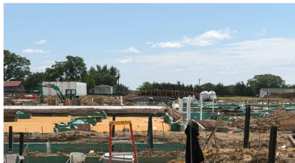
FOUNDATION & UNDERGROUND UTILITIES
