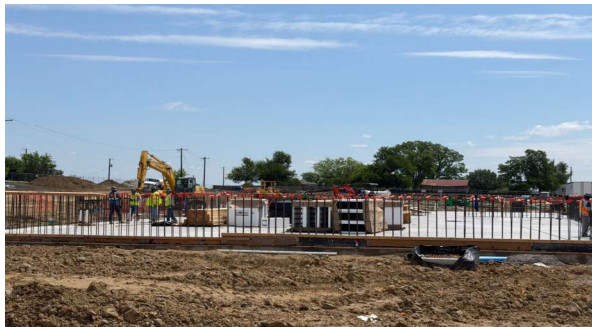
FOUNDATION & ICF REINFORCING
