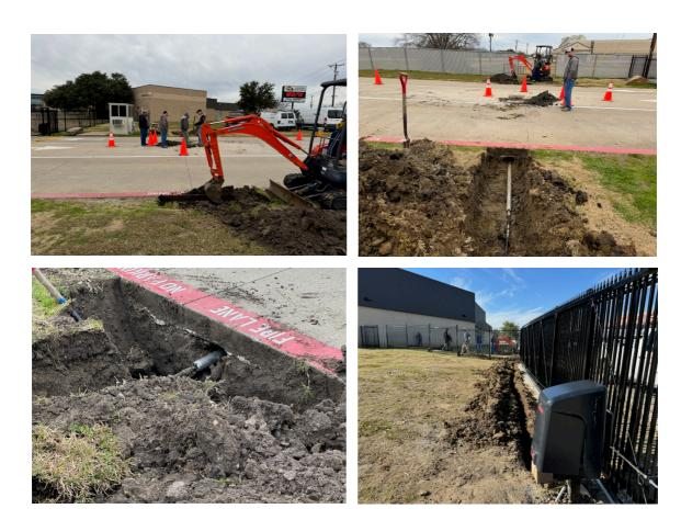
After a few cold days, the access tunnels were completed and the conduit was put in place. The table is now set for all the lines to be connected. The access controls on the security gates will be fully functional soon. Pictured below are guys from the team cutting through the concrete near the guard shack at the high school.
