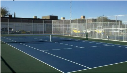
New Tennis Courts
