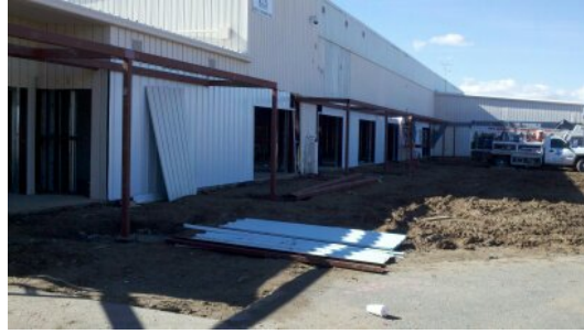
Metal Siding Repairs
