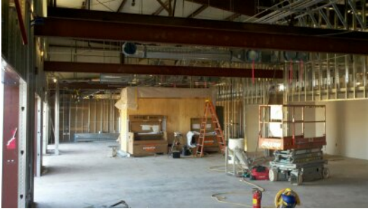
Framing and Drywall Installation
