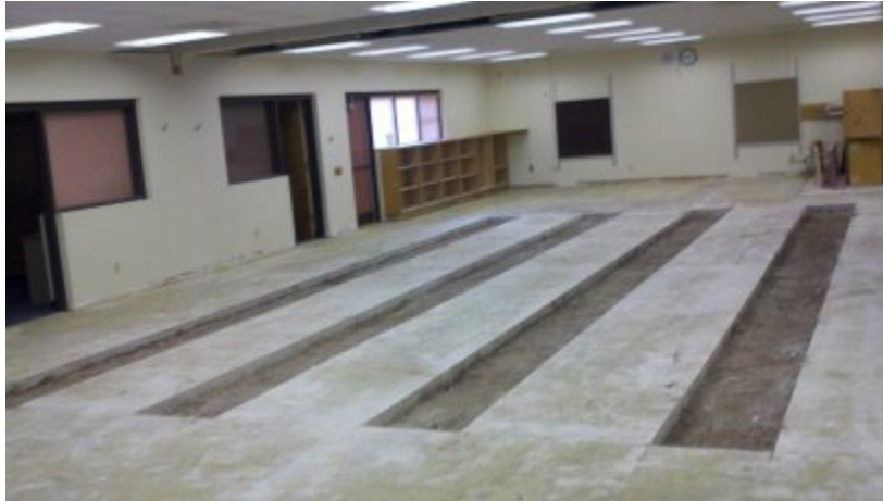
Classrooms 14 & 15 computer lab demolition
