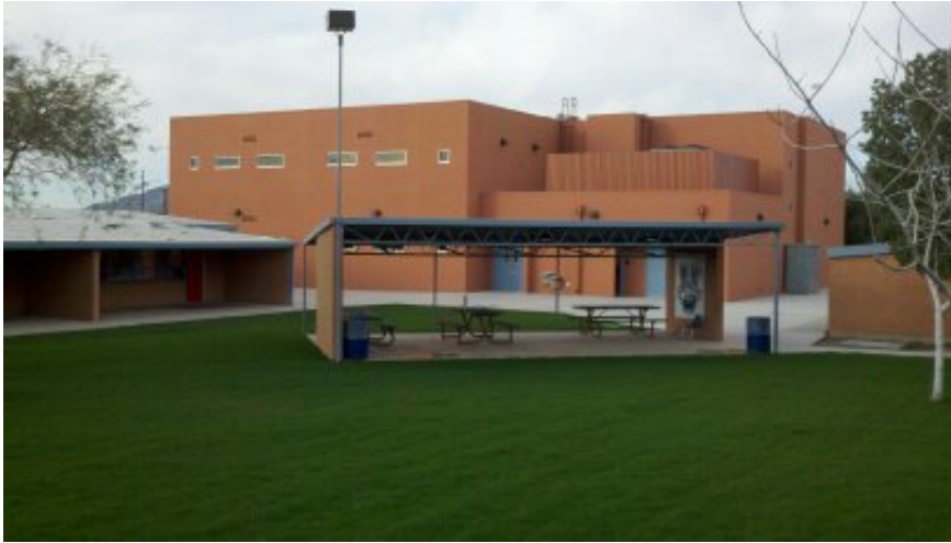
Nash 2 Story Classroom Building and Courtyard Repair
