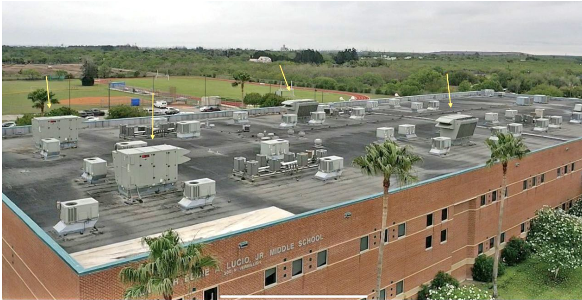
Lucio MS HVAC Upgrades
