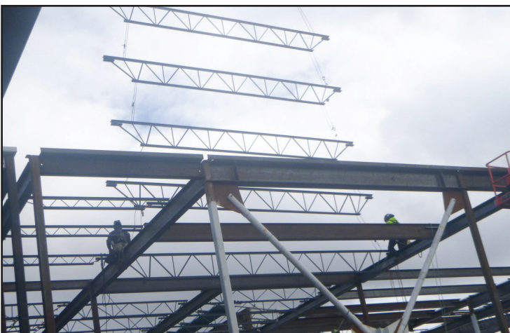
South wing roof
