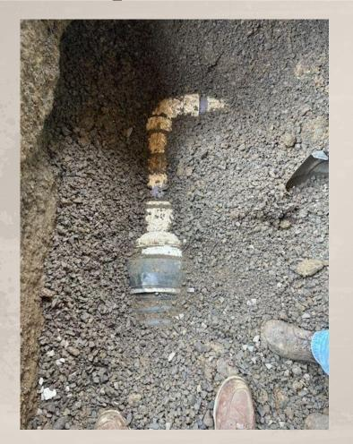
Connection from 4" downspout to the 12" trunk line
