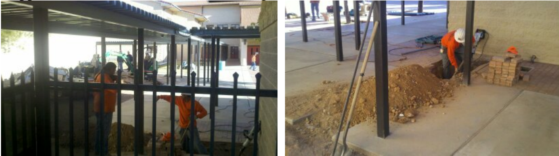
Underground Backbone Cable and Electrical Infrastructure Installation During Rodeo Break
