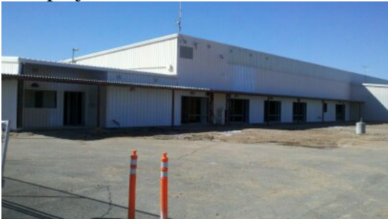
New Transportation Office Entry
