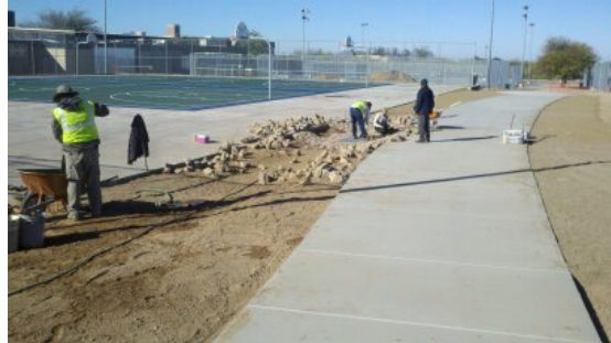
New Pedestrian Walkway from West Parking Lot to Stadium
