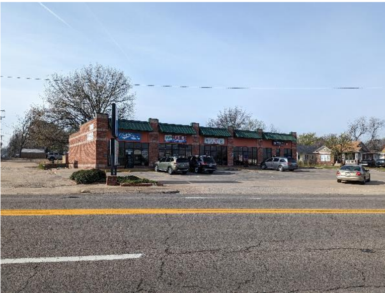
View of the south adjoining property beyond Rogers Avenue occupied by a strip mall.
