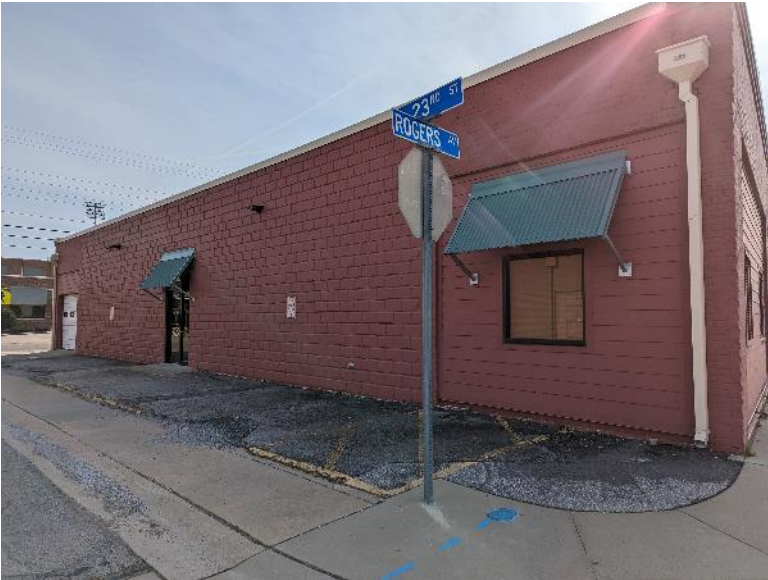
View of the west adjoining property occupied by the Fort Smith School District.
