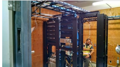
New IDF room addition
