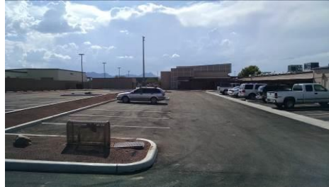
East Parking Lot
