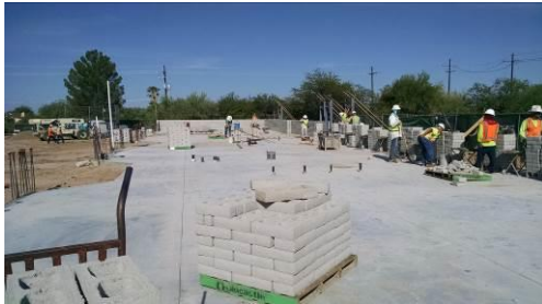
Walls being constructed for new classrooms
