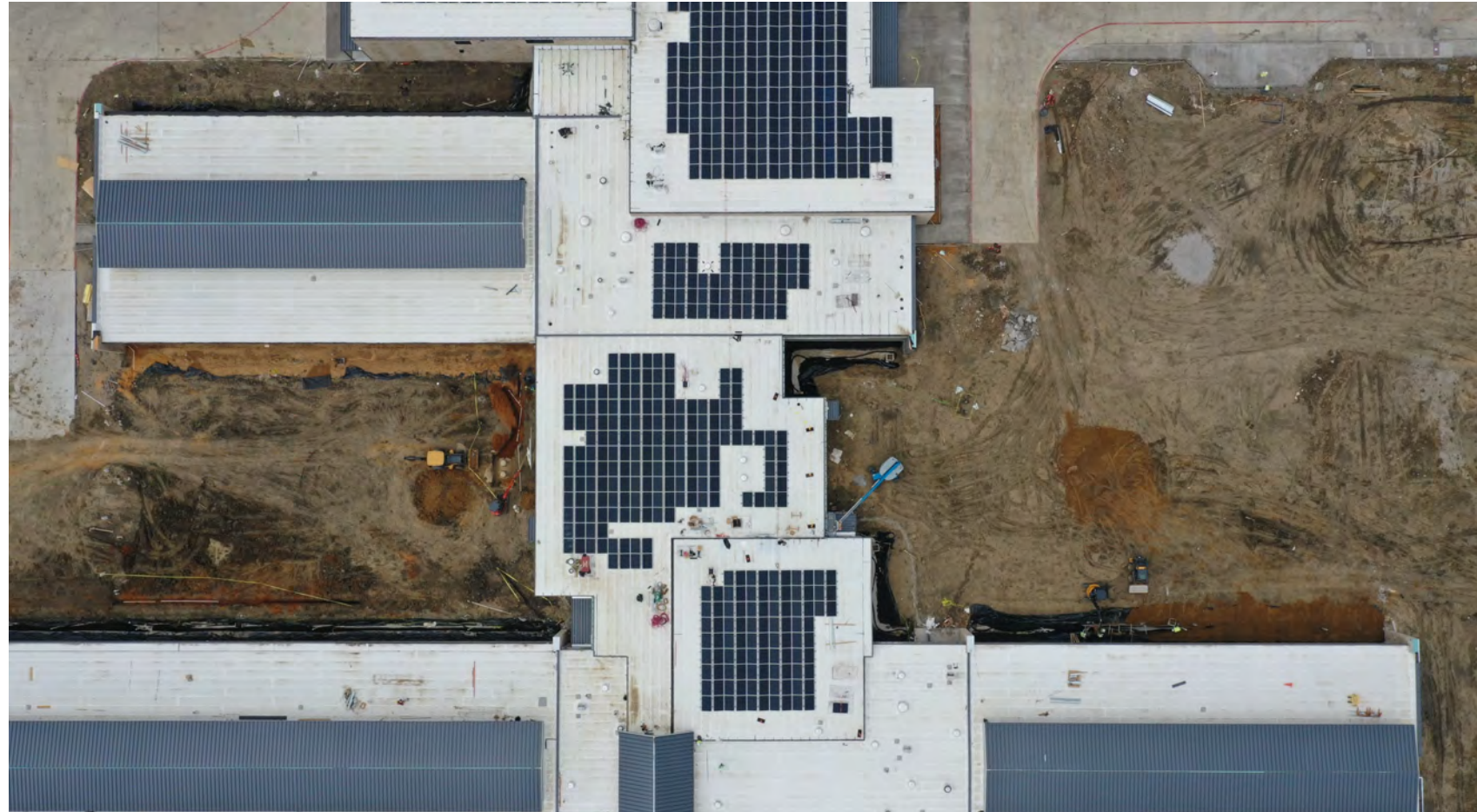
SOLAR PANEL OVERHEAD AERIAL VIEW
