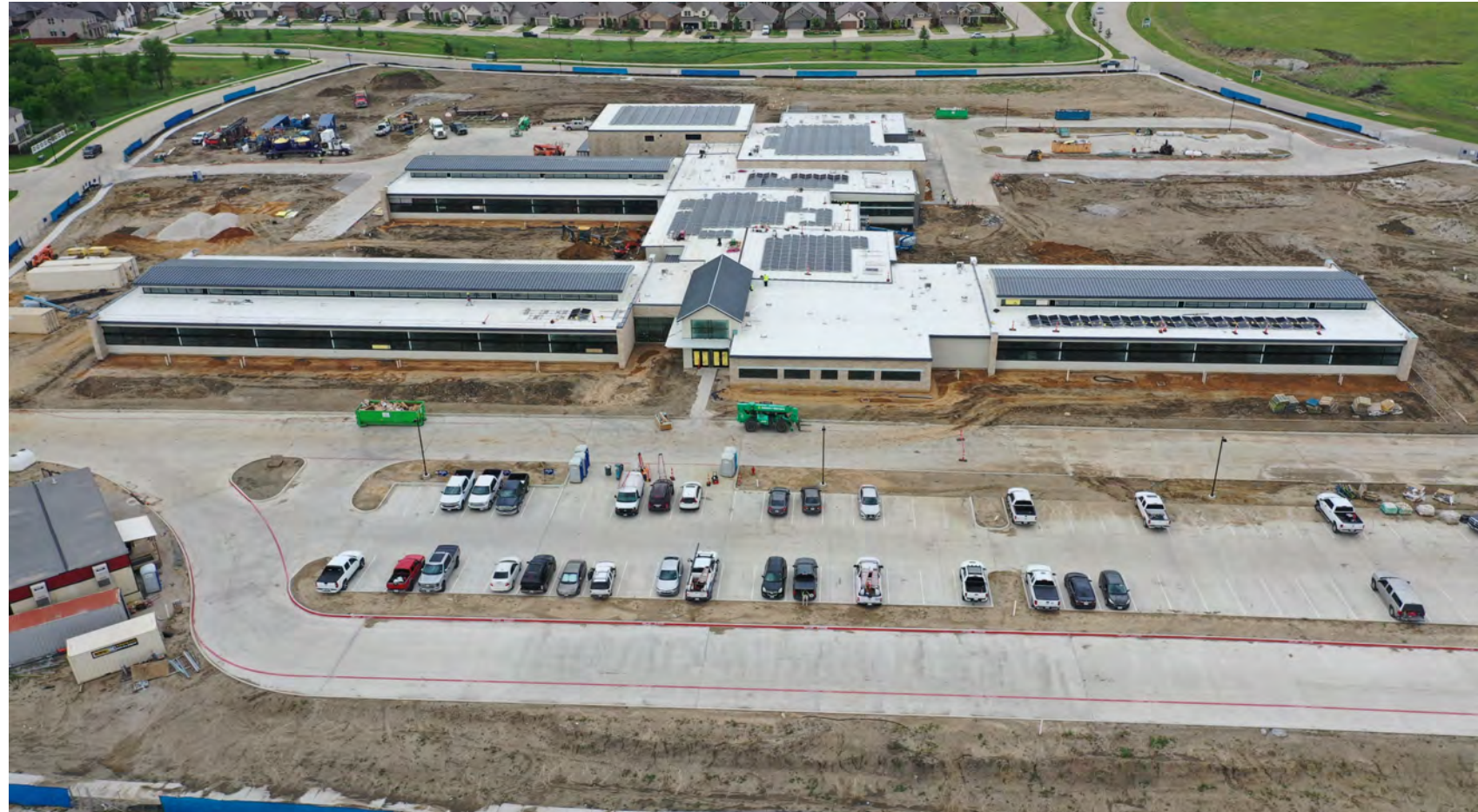
SITE VIEW LOOKING NORTH
