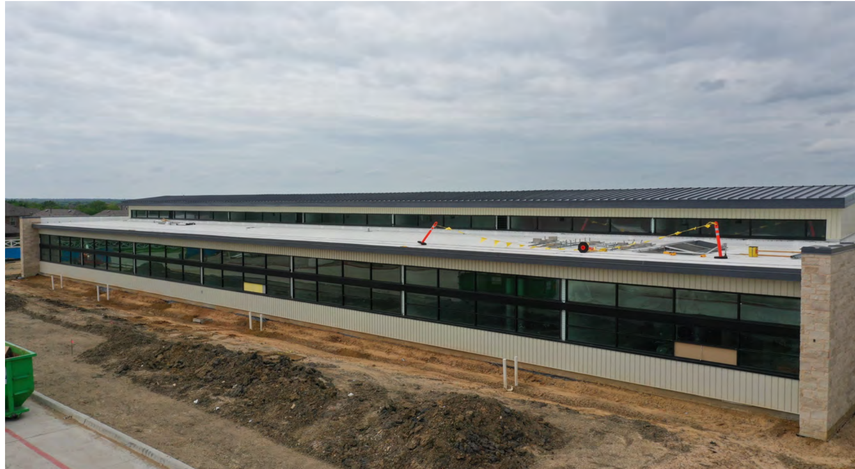
EXTERIOR CLASSROOM VIEW LOOKING NORTHWEST
