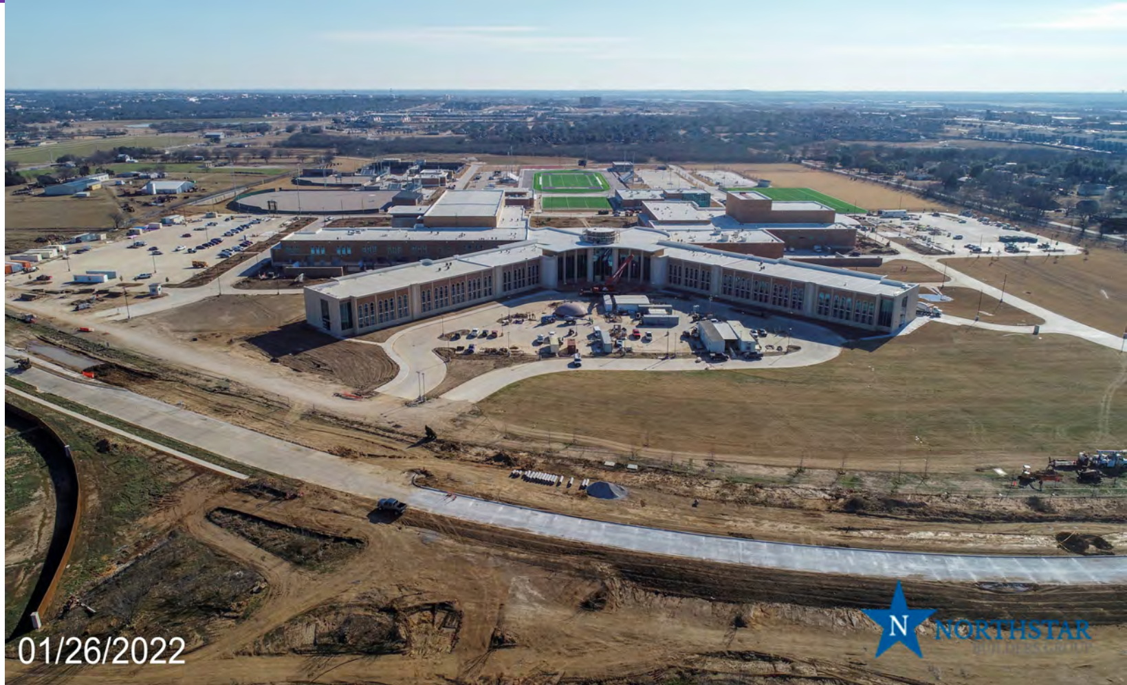
MAIN CLASSROOM BUILDING
