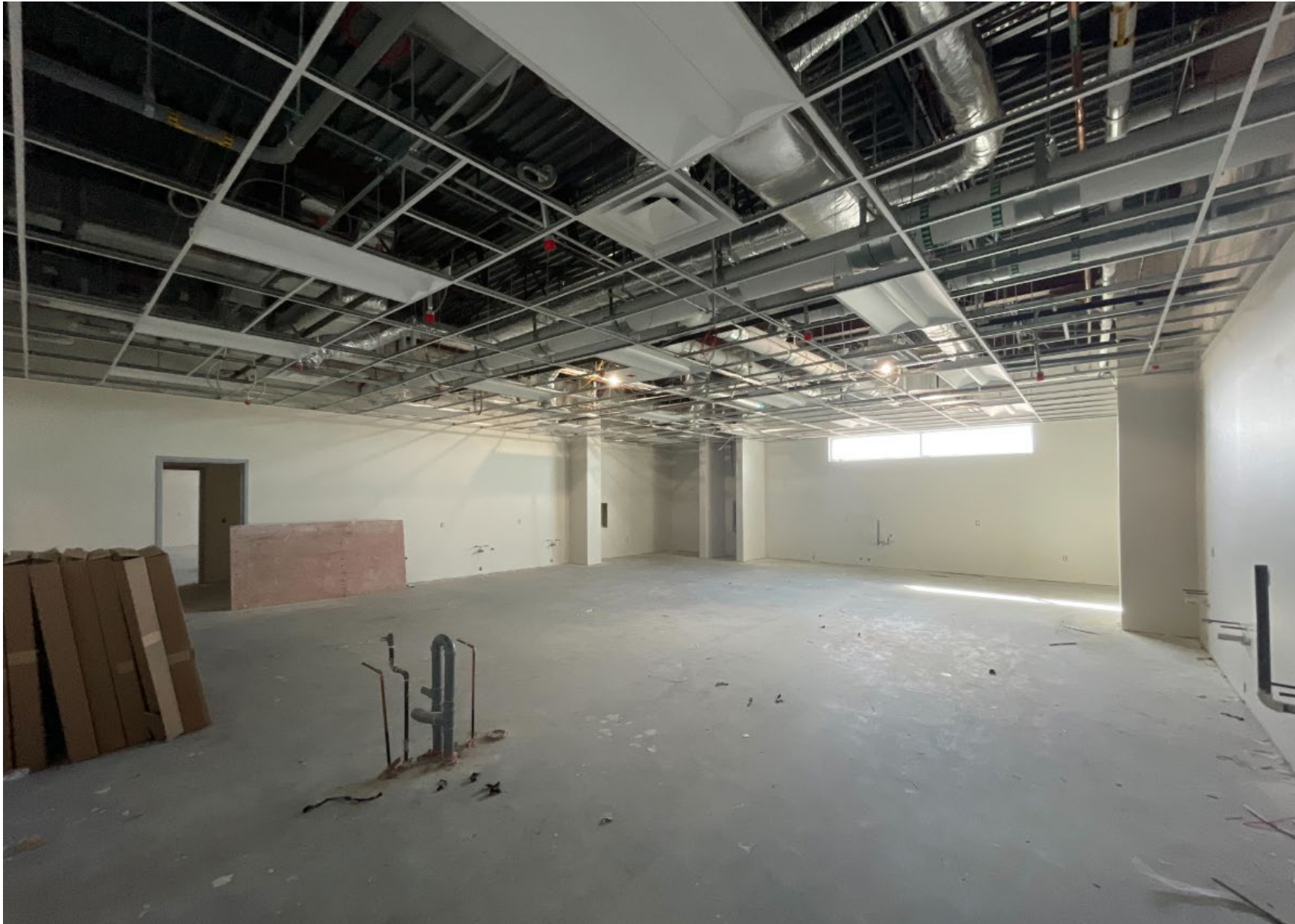
Classroom Wing Area A/A1
