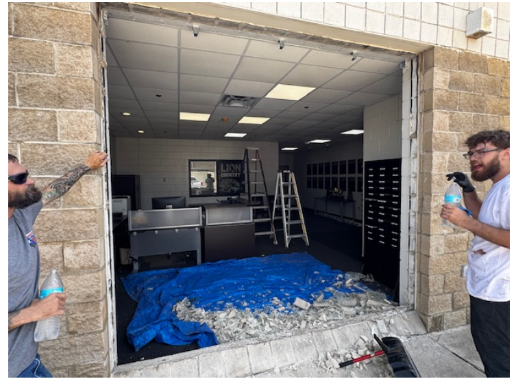
The front window at the field house was also replaced. The wall of glass blocks was removed and a new storefront style glass was installed. It looks much better!
