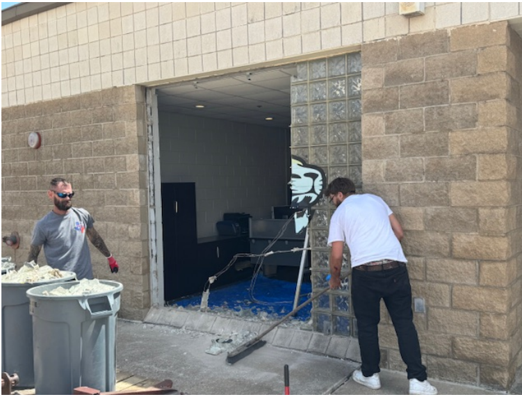
The front window at the field house was also replaced. The wall of glass blocks was removed and a new storefront style glass was installed. It looks much better!
