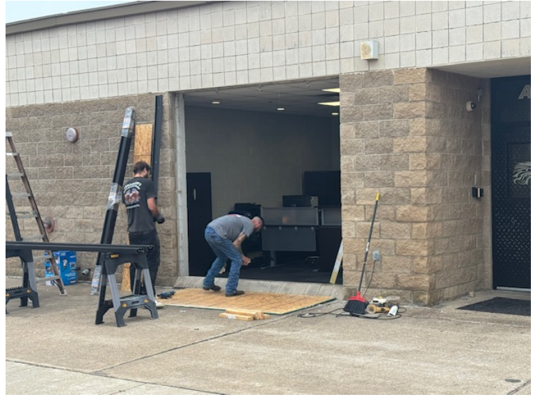
The front window at the field house was also replaced. The wall of glass blocks was removed and a new storefront style glass was installed. It looks much better!
