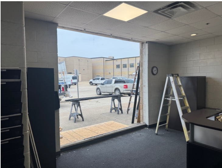
The front window at the field house was also replaced. The wall of glass blocks was removed and a new storefront style glass was installed. It looks much better!
