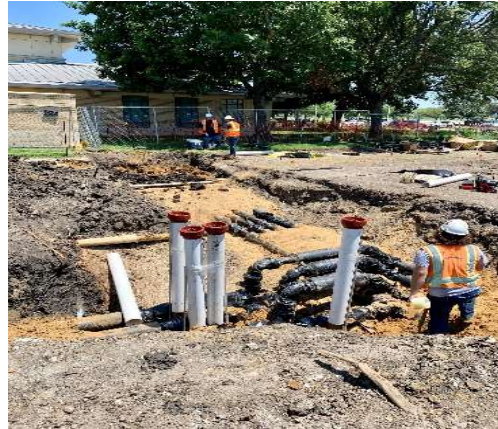
Install of Hydronic Pipes at Fire Lane
