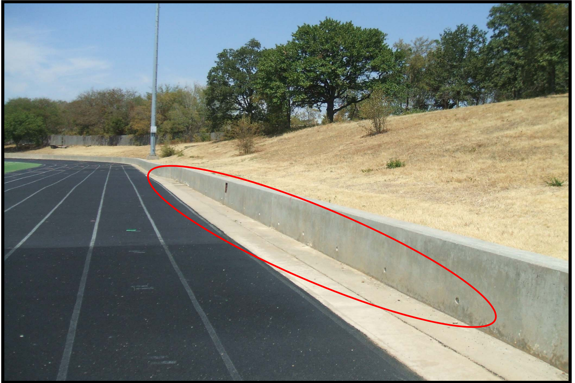
Weep holes in retaining wall drain across track
