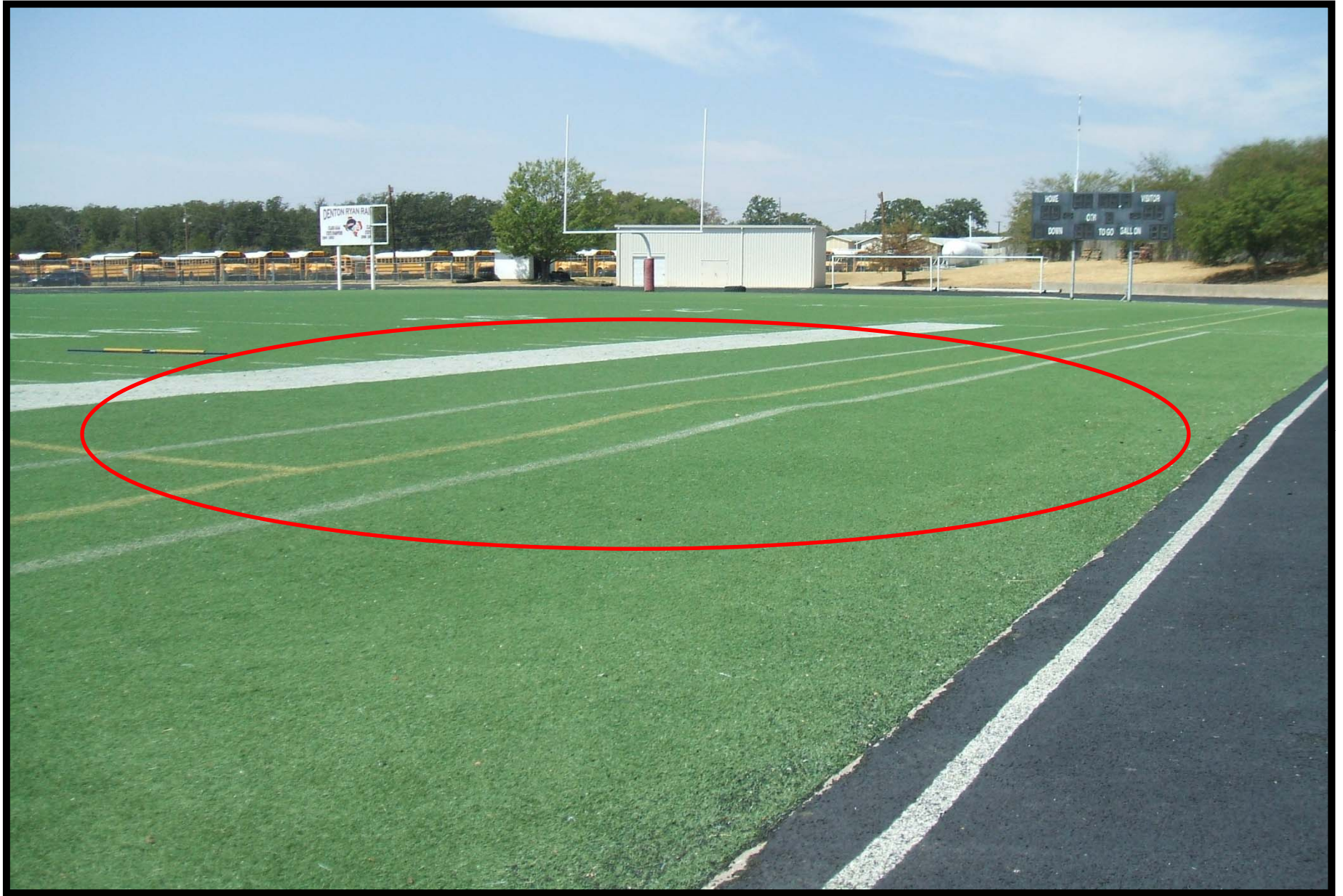
Uneven playing surface
