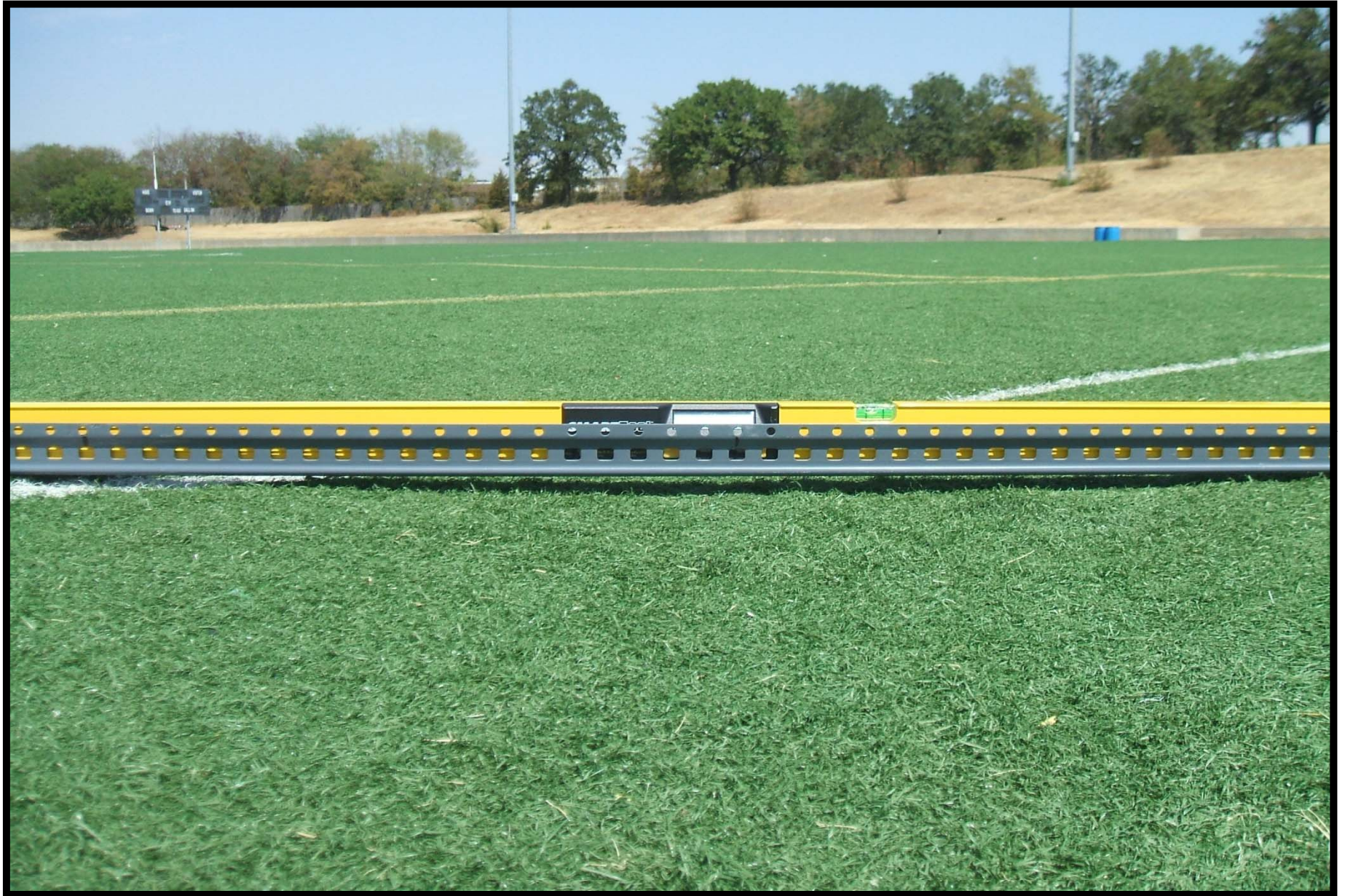
Movement in subgrade
