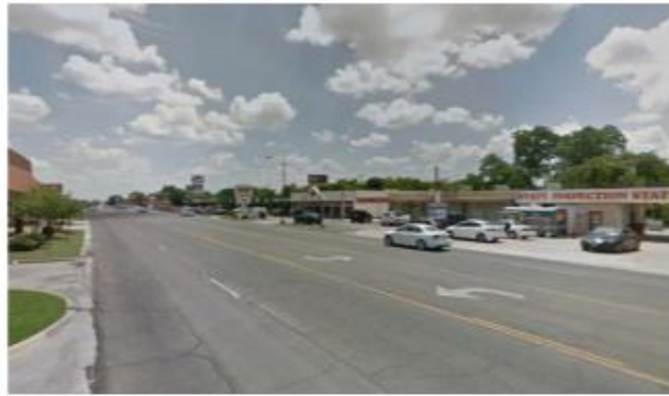
02 Signs Excessive signage creates visual clutter along the 31st Street corridor. The use of consolidated signs or enhanced construction materials could help improve the quality of the corridor.
