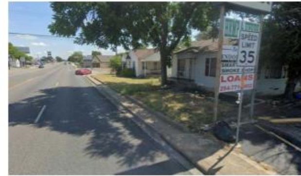
01 Sidewalks Narrow sidewalks that are frequently interrupted by driveways create unsafe conditions for pedestrians and decrease the walkability of this neighborhood.
