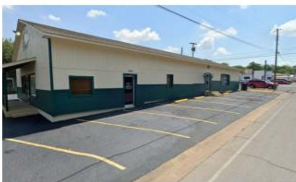
01 Parking along Corridor
