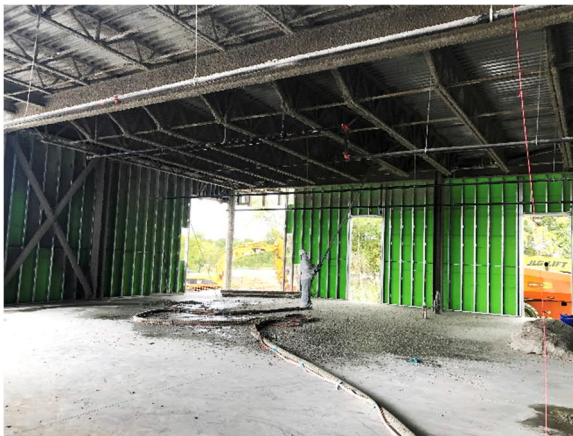
Fireproofing at the Student Center
