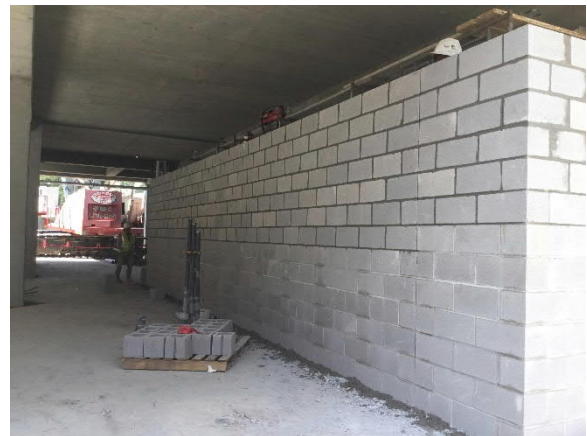
CMU Installation in Garage
