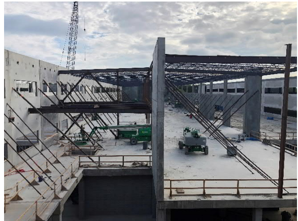
Steel Erection at Trade Bar C
