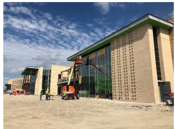
Southeast View of Masonry at the Library
