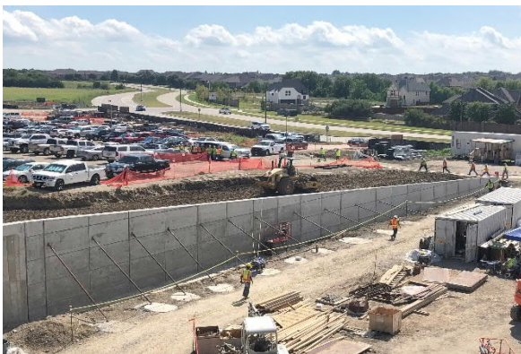
South Garage Entrance, Retaining Wall
