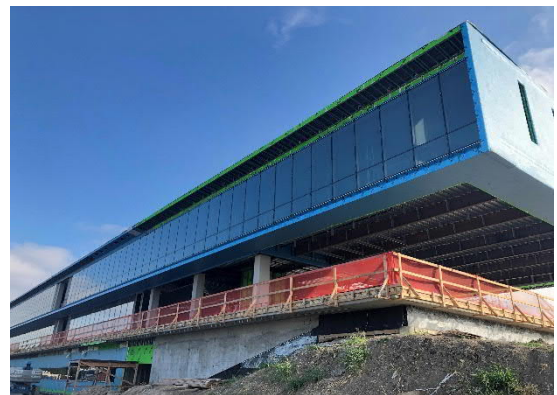
Windows Installed on South End of the Academic Building
