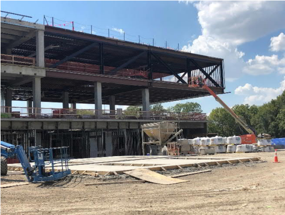
North Steel Truss on Academic Building
