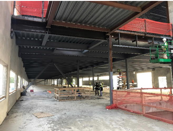
Steel Painted at Trade Bar B
