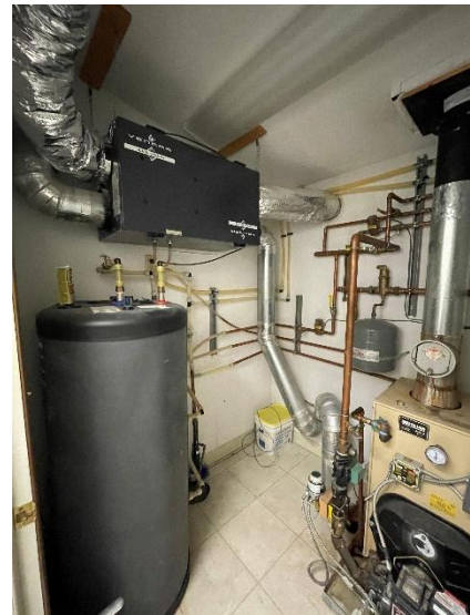
Photo M19 – Boiler Room
