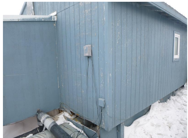
Photo E4– Typical Telephone Service NID
