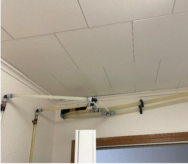
Photo M17– Exposed Pex Piping
