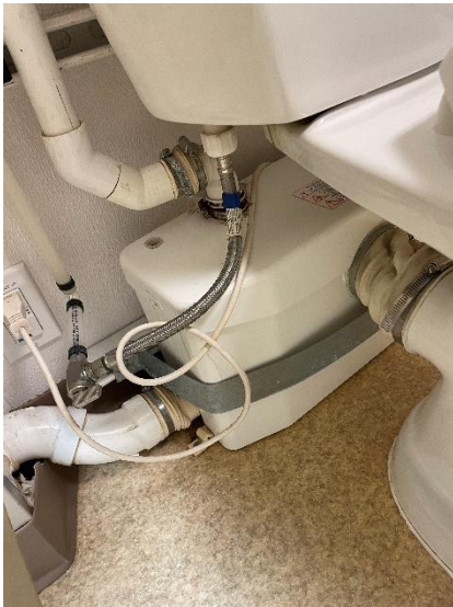
Photo M1 – Toilet and Lift Station
