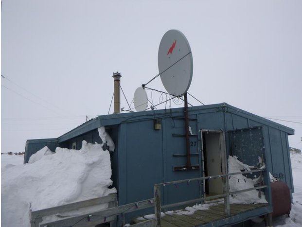
Photo E5 – Typical Satellite Dish
