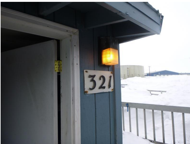
Photo E3 – Typical Exterior Lighting
