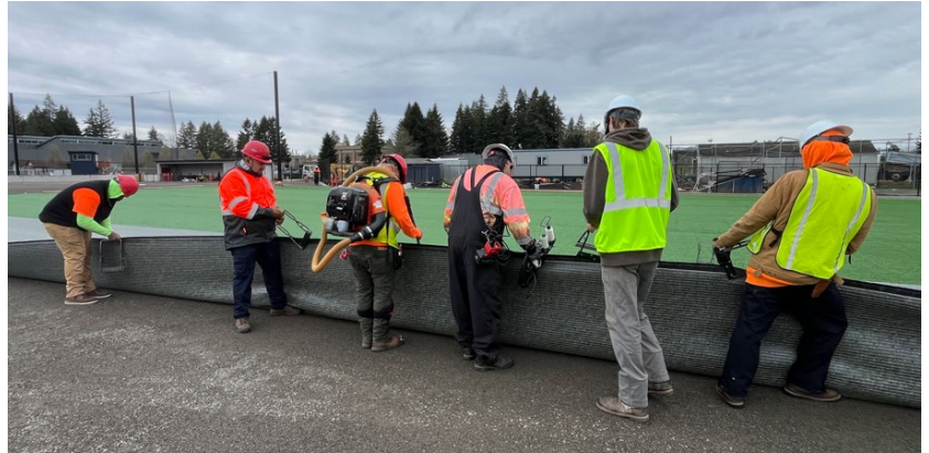
Softball dugout and turf installation
