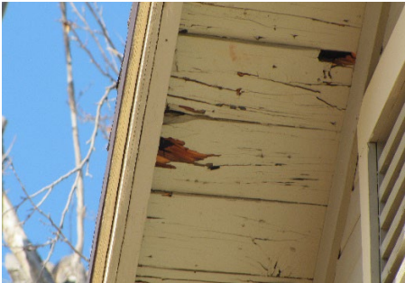
Eaves over vents at roof peak
