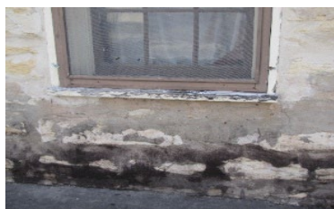
back building windows
