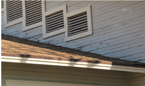
so. side siding and vent framing
