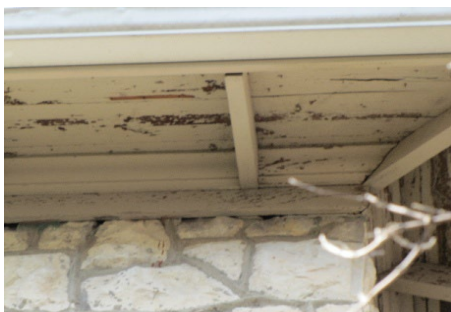
n/e corner eaves
