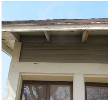
Eaves and fascia
