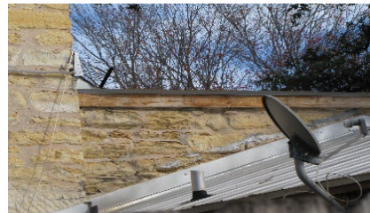
back of building
