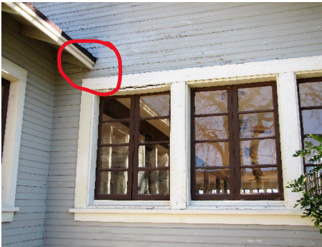
so. side kick out flashing
