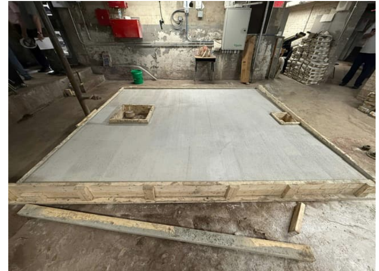
CONCRETE PAD FOR NEW BOILER
