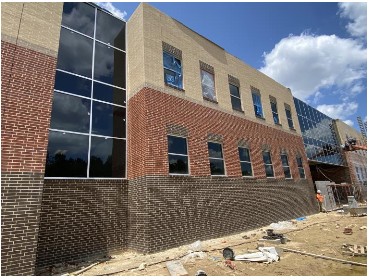
Curtain Walls Installed on the East Side
