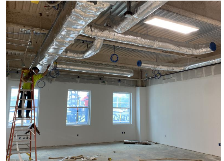
Ductwork Insulation on 2 nd Level
