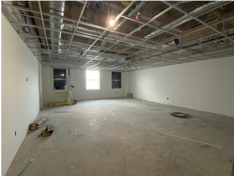
Ceiling Grid Installed on 2 nd Level
