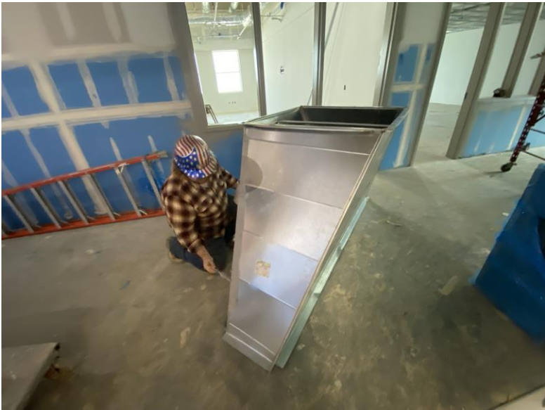
Installing Ductwork on 1 st Level
