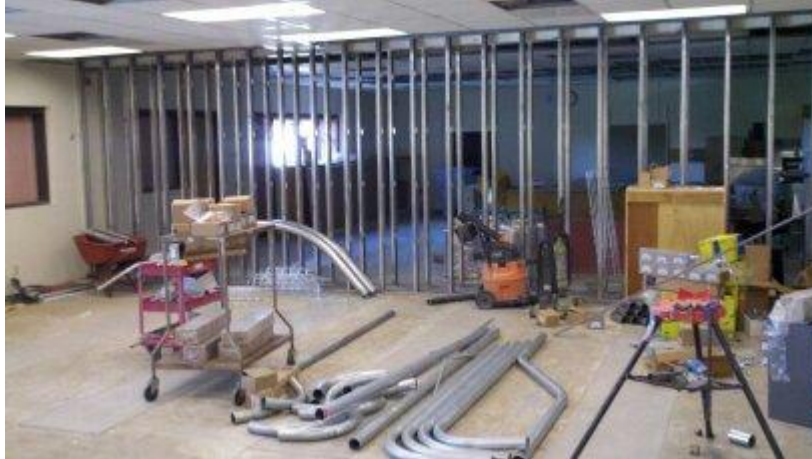
Copper Creek Classrooms 14 & 15 computer lab construction
