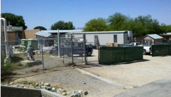
CDO Construction Lay-Down Yard
