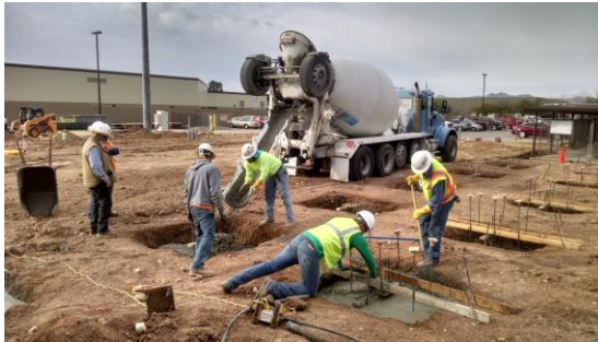
Professional Development Building Footer Installation
