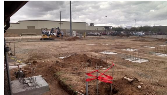
Professional Development Building Footer Installation
